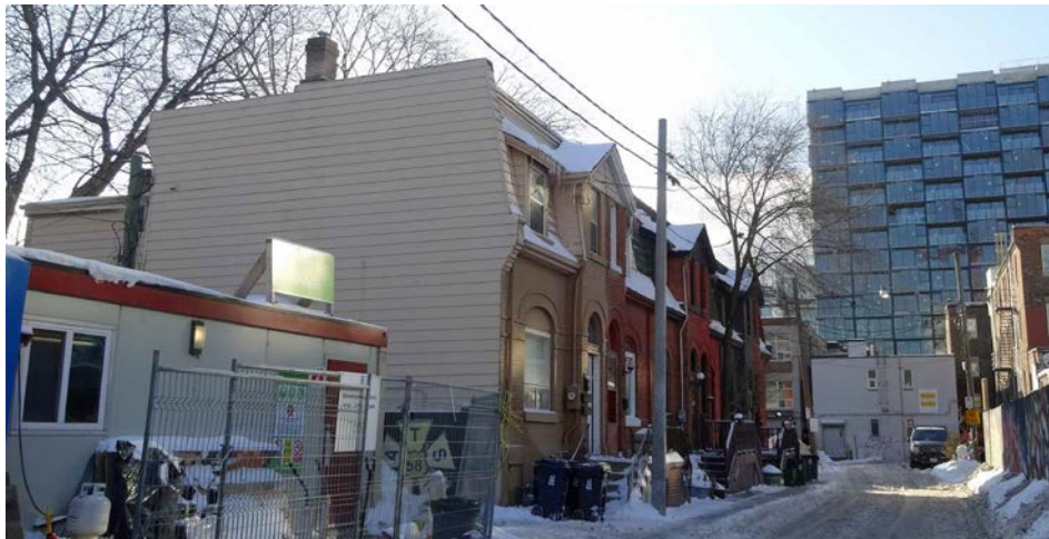
Above: 1-11 Adelaide Place looking south from Adelaide Street West toward Waterloo Terrace; cover: west elevations of the William Clarke Row Houses (Heritage Preservation Services, 2015)
