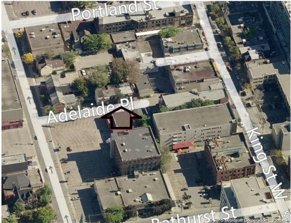
15. Current Photograph, 1-11 Adelaide Place, 2015 : looking east and showing the William Clarke Row Houses on the east side of the street south of Adelaide Street West (left) with the adjoining mixture of residential and industrial buildings ( www.bing.com/maps )
