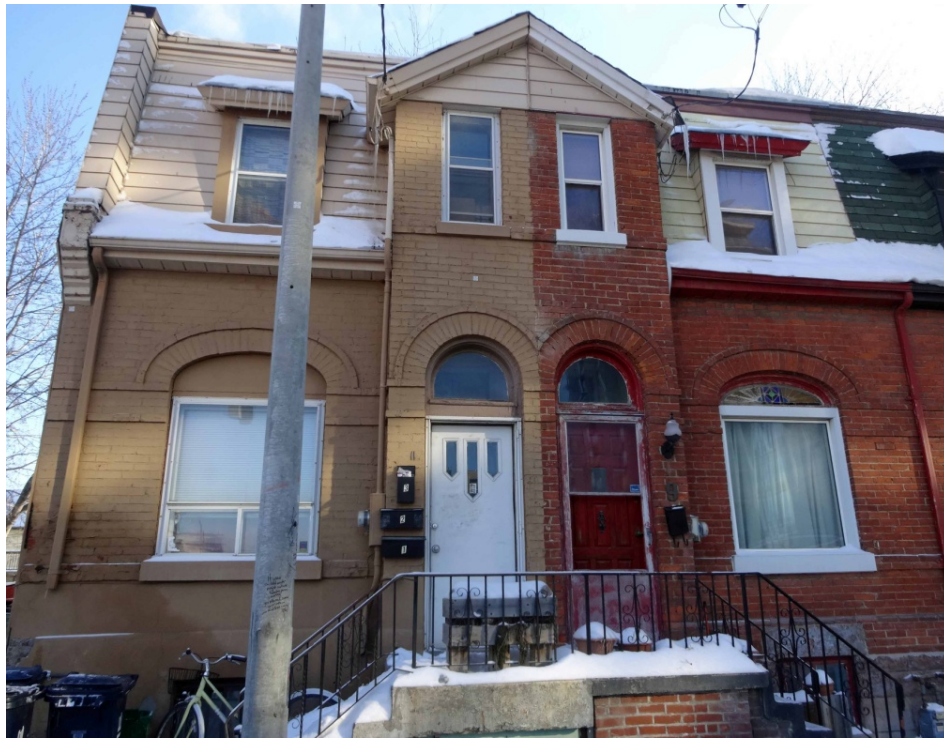
14. Current Photographs, 1-11 Adelaide Place, 2015: showing the row houses at 5-7 Adelaide Place (above) and 9-11 Adelaide Place (below) (Heritage Preservation Services)
