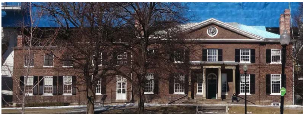
35. Current Photographs, The Grange and Grange Park, 2015 : showing the south elevation of The Grange with one of the commemorative plaques (above) and the location and setback of the west wings dating to the 1840s (centre) and 1885 (left) (Heritage Preservation Services)
