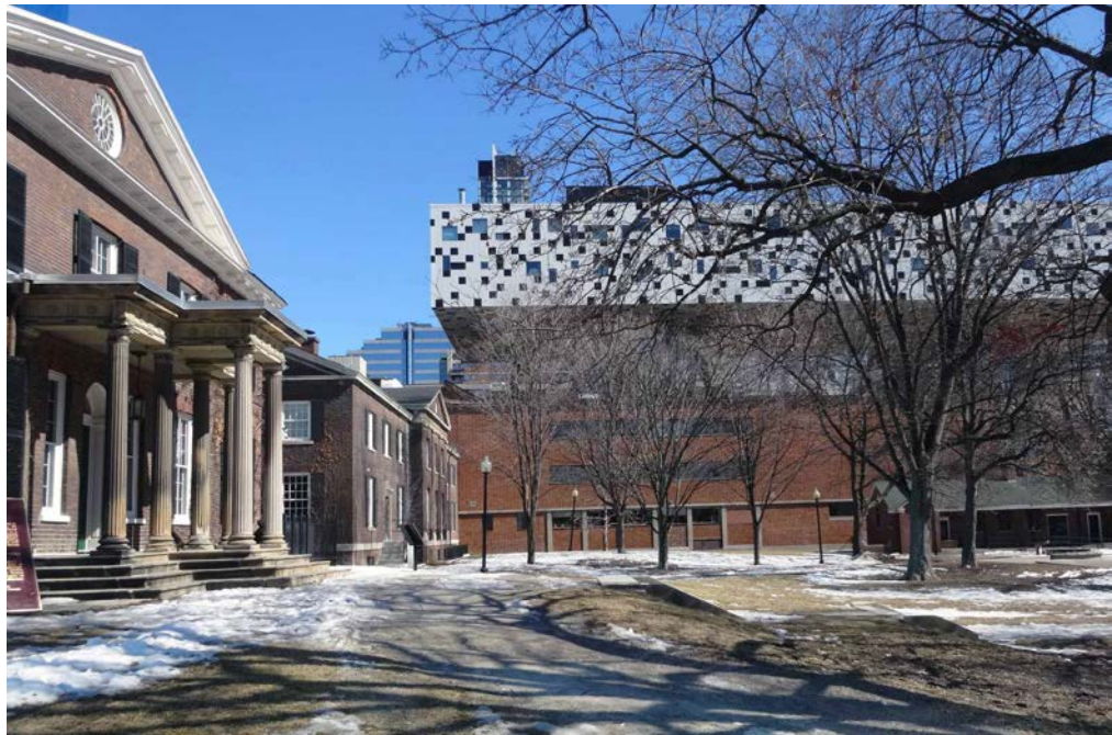
36. Current Photographs, The Grange, 2015 : showing the west wings of The Grange dating to the 1840s (right) and 1885 (left) (above), and the raised setting of The Grange adjoining the semi-elliptical-shaped driveway (below) (Heritage Preservation Services)
