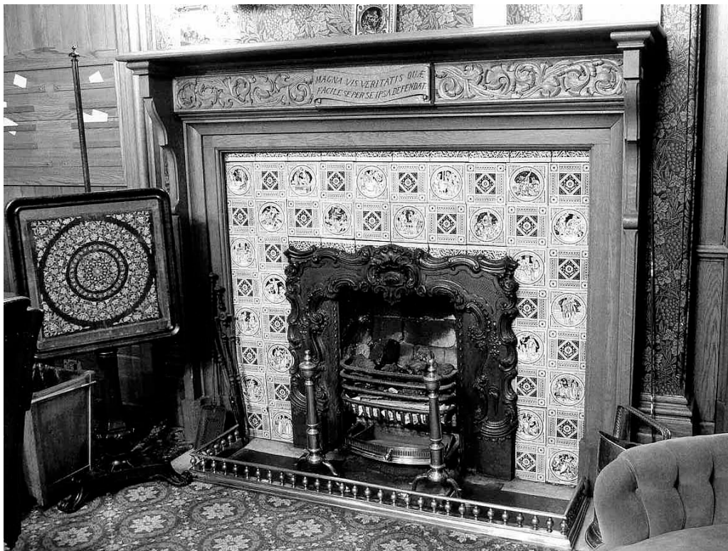
34. Interior Photographs, The Grange, 2005 : showing the Library in the west wing (1885) with the ceiling mouldings, the wood paneling, the paneled wood doors, the door and window trim, and the fireplace with the mantel and the tiled surrounding depicting scenes from Shakespeare's plays (Heritage Easement Agreement)
