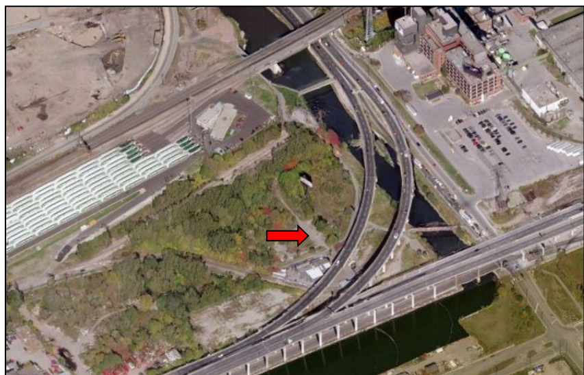
FIGURE 4: Location of Existing Third Party Ground Sign
