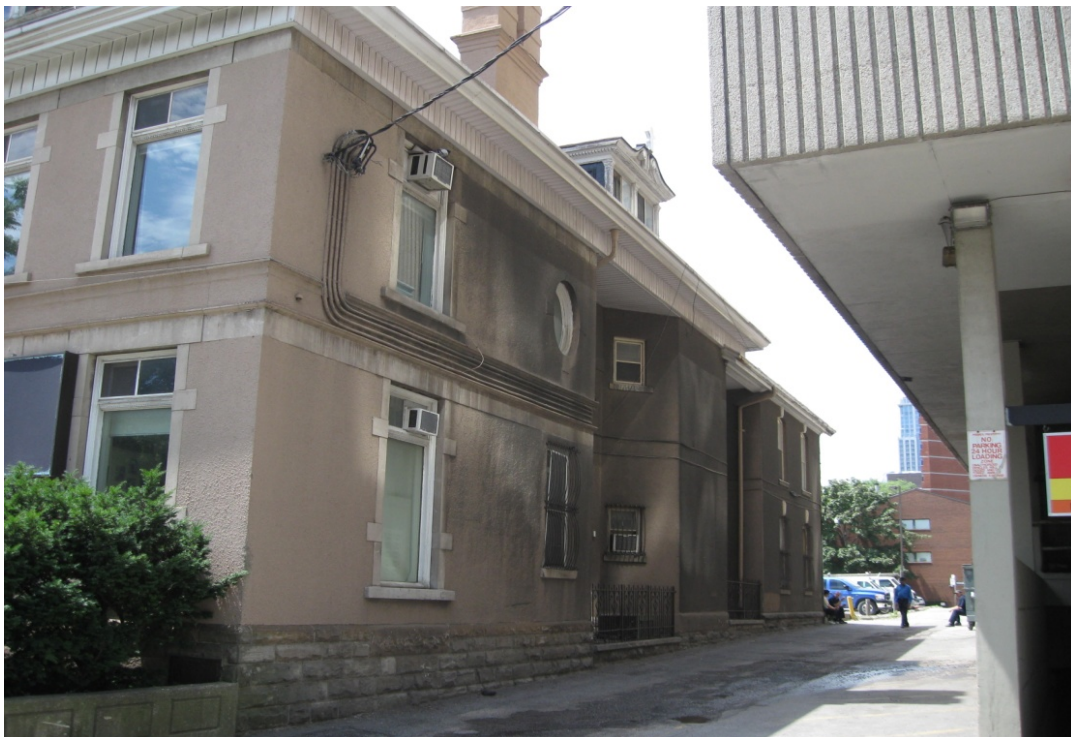
View of northeast corner
