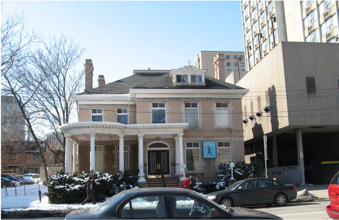
View looking west – main elevation
