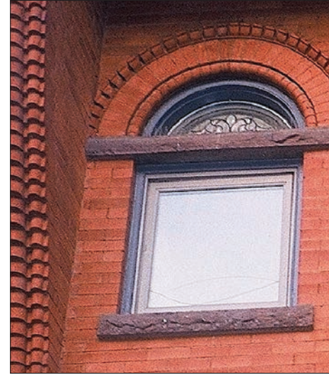
Annex Style details--specialty terra cotta and brickwork, rusticated stone lintel and sill, roundheaded window with stained glass
