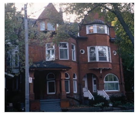
(above) Example of a Centre Hall Rotated Asymmetric Semi detached on Madison Avenue, note side entrance
