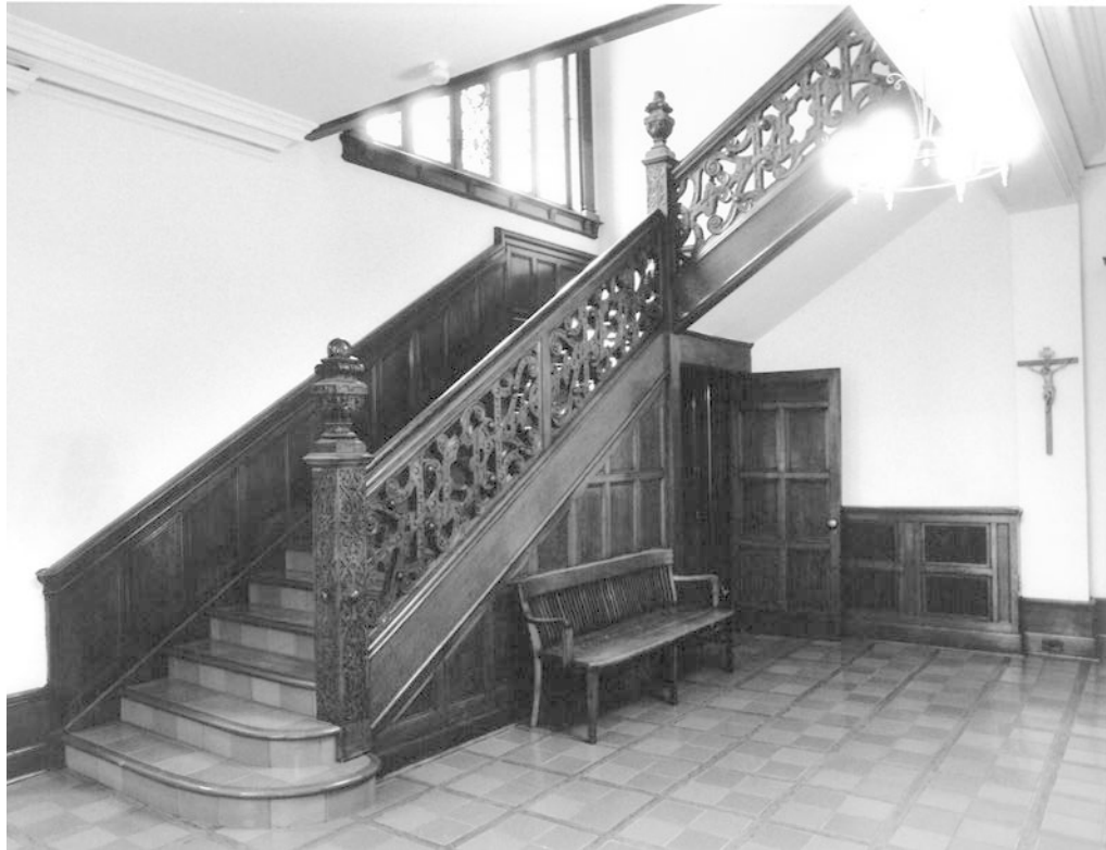
58. General view of the Entrance Hall : Showing the wood paneling, the quarter-turn staircase with a landing and the stair hall window. ( Photograph 16 , HEA )
