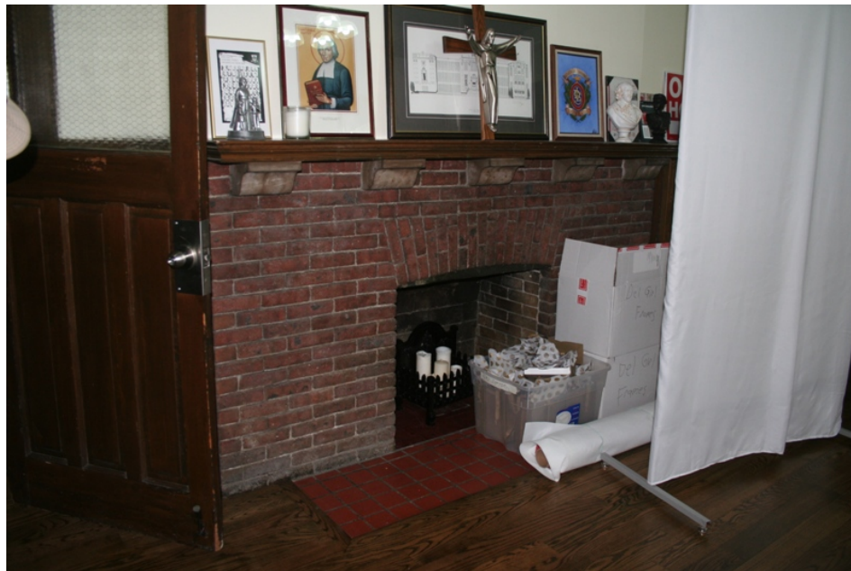
57. Dining Room Fireplace: Showing the brick fire surround with stone corbels supporting a wood mantel. The character of the fireplace completes the character of the room with its wood beamed ceiling and flattened Gothic Revival arches. This fireplace is not included in the HEA. ( HPS, 2015 )
