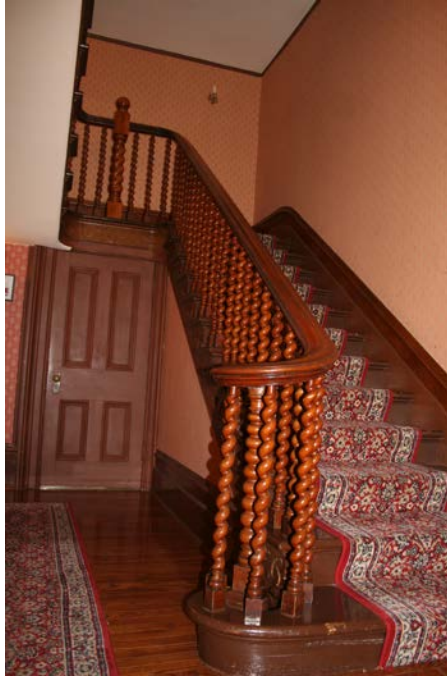
65. General view of the two-turn open well staircase: Showing the second storey as it rises to the third storey with twisted balusters. Included in the HEA, Photograph 21. (HPS, 2015)
