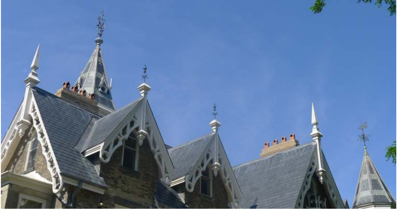
39. Oaklands, West Wing, 1869-70, Bargeboards and Finials and Weathervanes : Showing the south-west corner with the weathervane of the 1859-60 house at far-right. (HPS, 2015)
