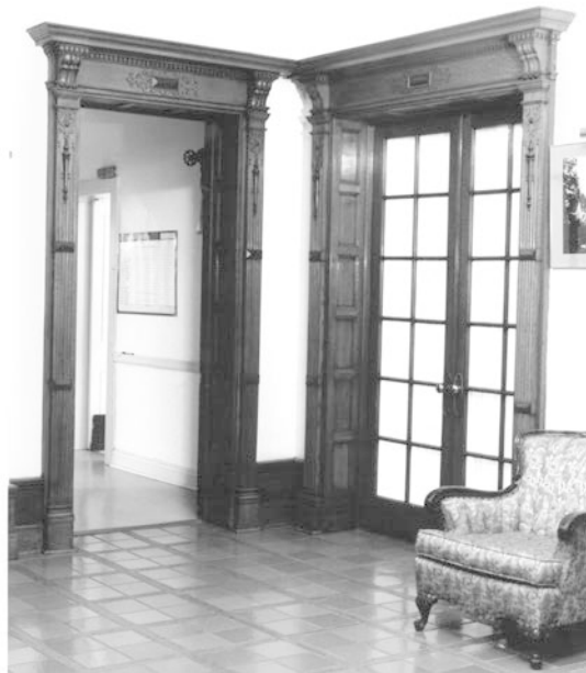
49. Main Entry Vestibule view of two door cases: Showing two Neo-classical door cases with fluted pilasters supporting entablatures with console brackets and cornices. ( Photograph 10, HEA )
