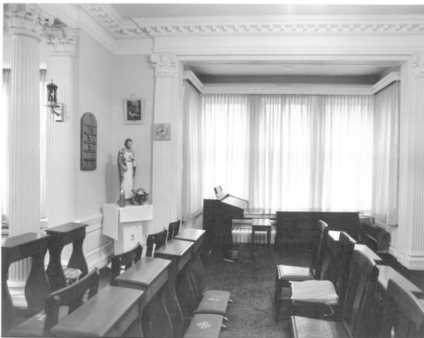
52. View of the south-west corner of the Chapel: Showing the bay window, fluted Corinthian pilasters, Corinthian columns and cornice. ( Photograph 12 , HEA )
