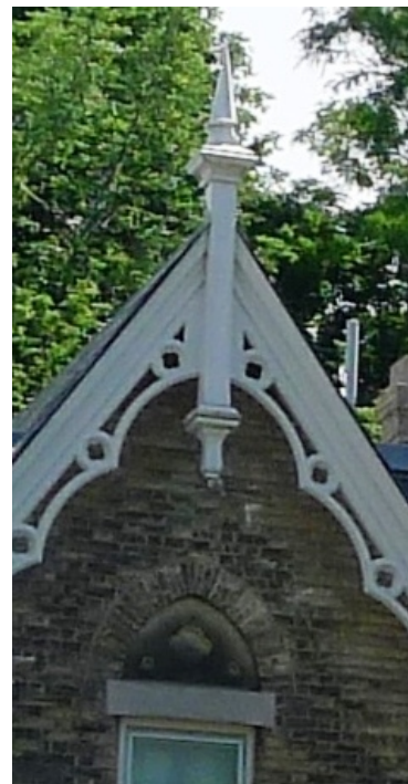
40. Oaklands 1869-70 Kitchen Wing (with c1912 wing at far left) (above left) : Showing Kitchen wing bargeboard patterns with simple scallop and quatrefoil motif. (HPS, 2015)
