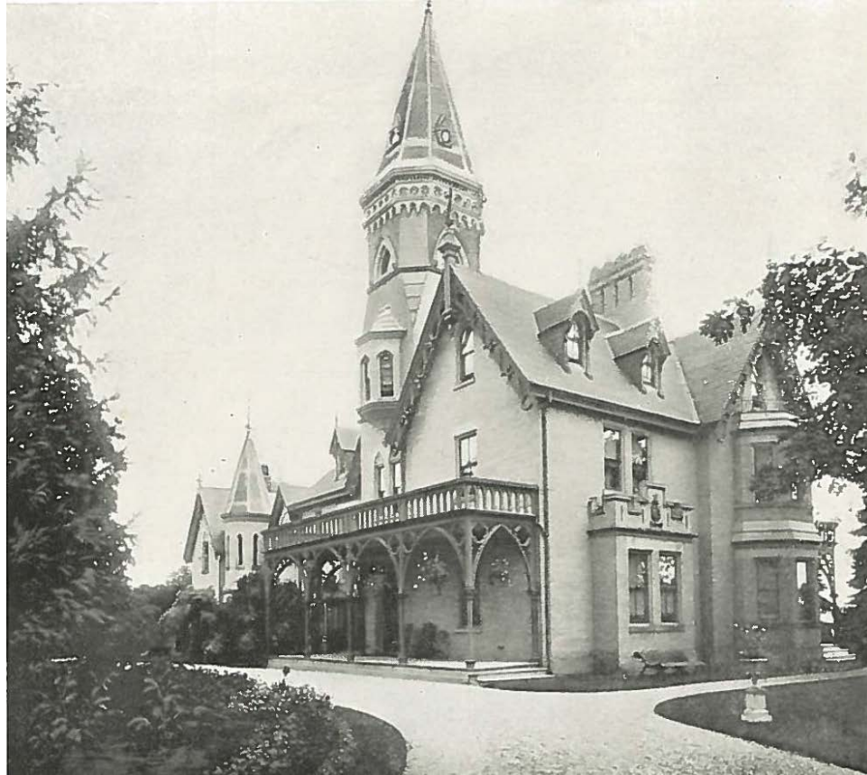
36. Oaklands, North-west Elevations, c 1896 : Showing the 1869-1870 additions by Gundry and Langley including the west wing with its bay windows, verandahs, and the 5-storey tower and beyond new kitchen wing and smaller tower. ( Engelhardt, p 26. )
