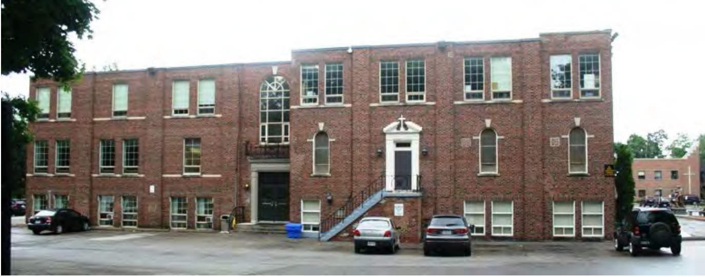
76. De La Salle College "Oaklands", north façade: Showing the façade that faces the approach from Farnham Avenue. The chapel is at right with white entry door case and three round-headed windows. Classroom wing is at the left with a stone framed entry and window with circular head and stone keystone. ( Heritage Preservation Services, 2015 )
