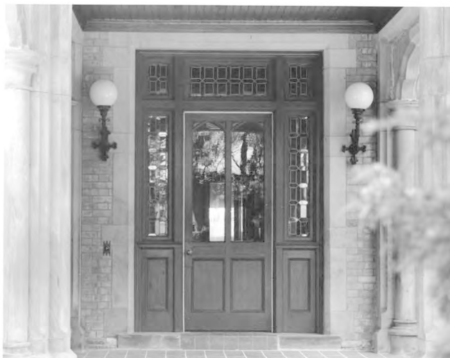
47. Main Entry: Showing the paneled door with two pointed-head lights, surrounded by a paneled door case containing multi-paned sidelights and a transom. ( Photograph 6, Heritage Easement Agreement (HEA) 1995 )
