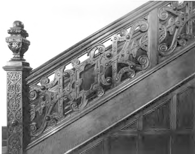
59. Detail of the Main Entry Hall staircase : Showing decorative wooden balustrade and the carved detailing of a newel post and cap. ( Photograph 17, HEA )
