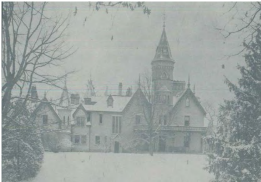
37. Oaklands, North Elevation, c 1905 : Showing the 1869-1870 additions by Gundry and Langley with the tower, gable wing at the right, and the smaller tower and one-and-a-half storey kitchen wing at the left of the photo. ( Canadian Archives, PA119997 )
