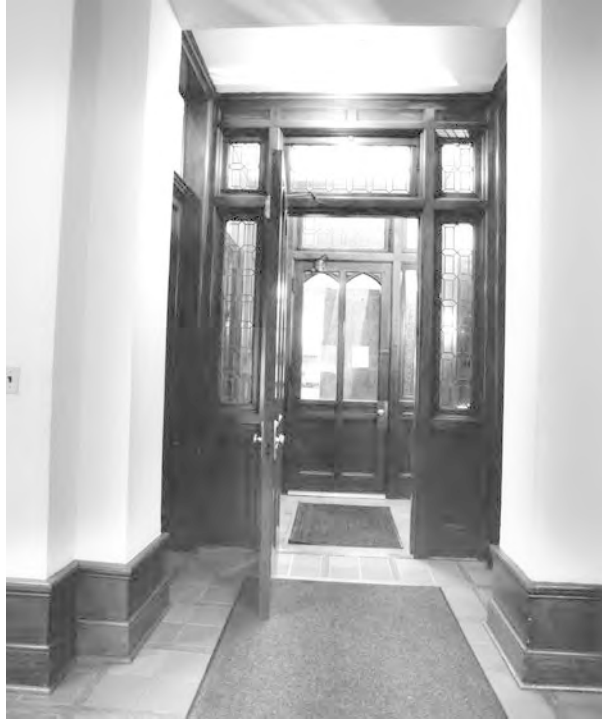
48. Interior View of Main Entry Vestibule: Showing the paneled door with two pointed-head lights, surrounded by a paneled door case containing multi-paned sidelights and a transom and matching internal screen. The glazing details match that of the staircase window. ( Photograph 9, HEA )
