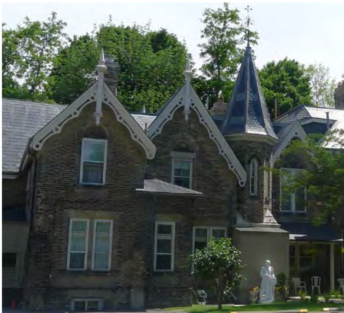
40. Oaklands 1869-70 Kitchen Wing (with c1912 wing at far left) (above left) : Showing Kitchen wing bargeboard patterns with simple scallop and quatrefoil motif. (HPS, 2015)
