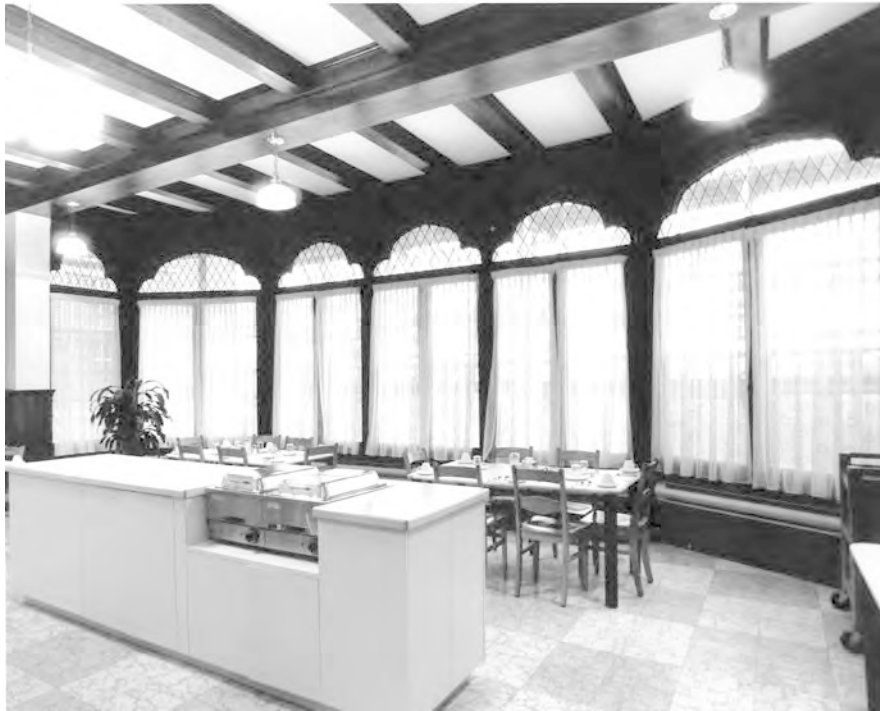
56. General view of the south wall of the Dining Room: Showing the wooden arcaded window with flattened Gothic Revival arches and wood ceiling beams. ( Photograph 15, HEA )
