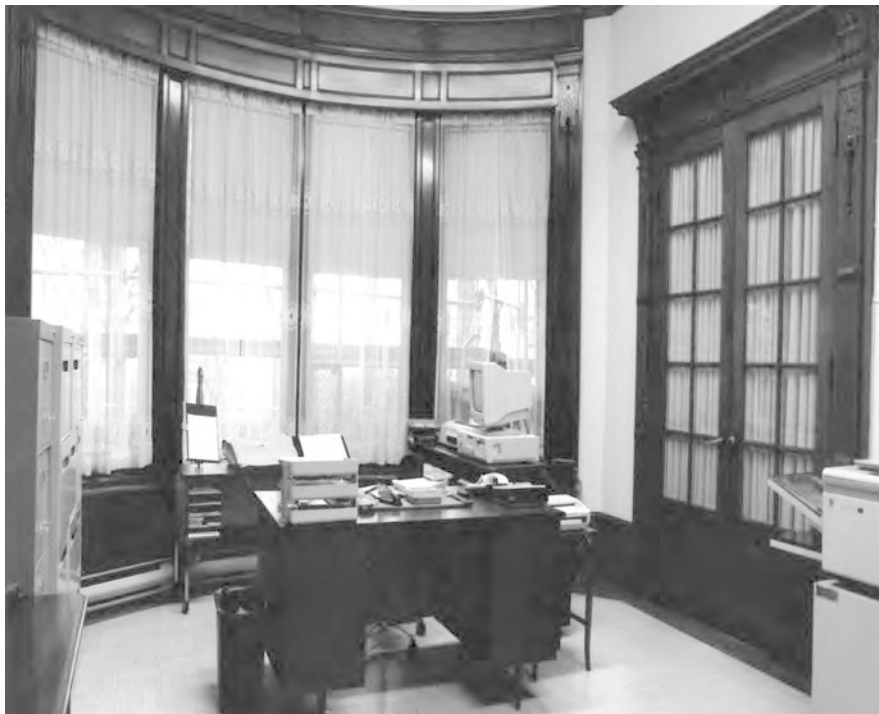
55. General view of the south wall of the office: Showing the bow window framed by wood paneling and the multi-paned double-doors with ornamented wooden surround. (Photograph 14 , HEA)
