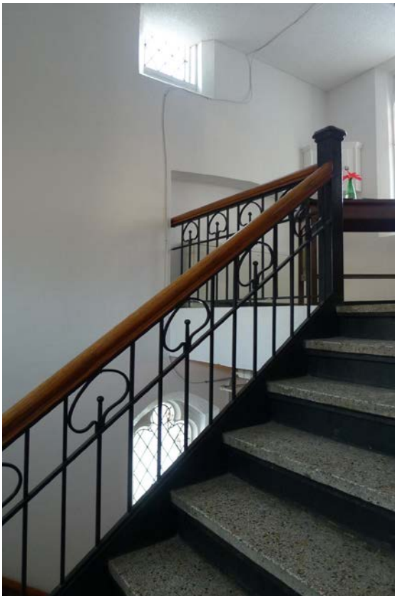
51. Church Staircase, Main Entry, 1931. ( Heritage Preservation Services, 2015 )
