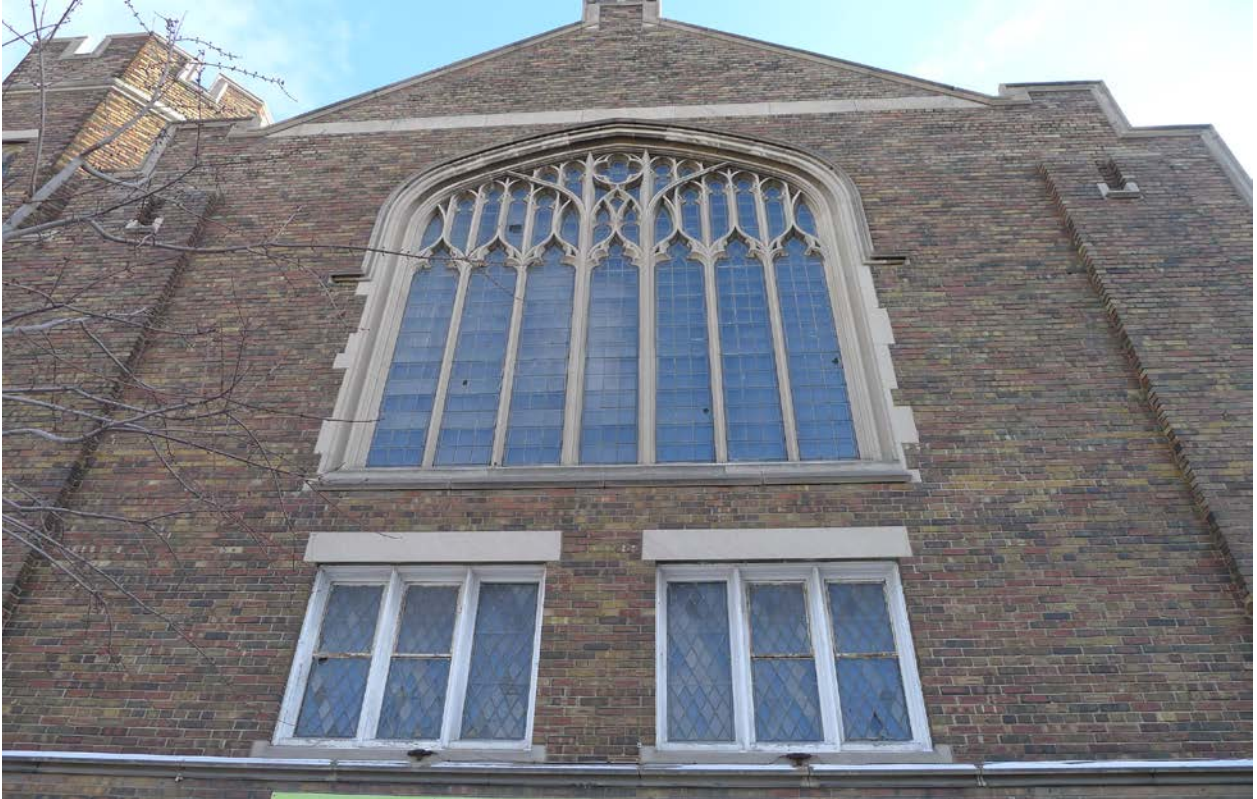
37. Church, North façade : showing stone traceried window and leaded glass, stone trim on parapet and belt course below windows. ( Heritage Preservation Services, 2015 )
