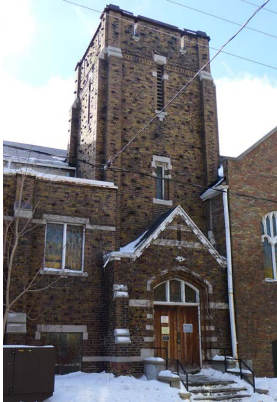
22. Sunday School, east elevations tower and entry details, 1911 : showing the combination of stone details especially around the doors, windows, buttresses and the gable of the entry porch. Note also the brick and stone details in the tower and the projecting bricks. ( Heritage Preservation Services, 2015 )
