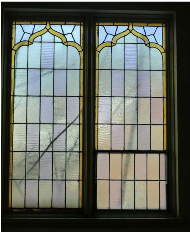
31. Sunday School Classroom, detail of leaded glass windows. ( Heritage Preservation Services, 2015 )
