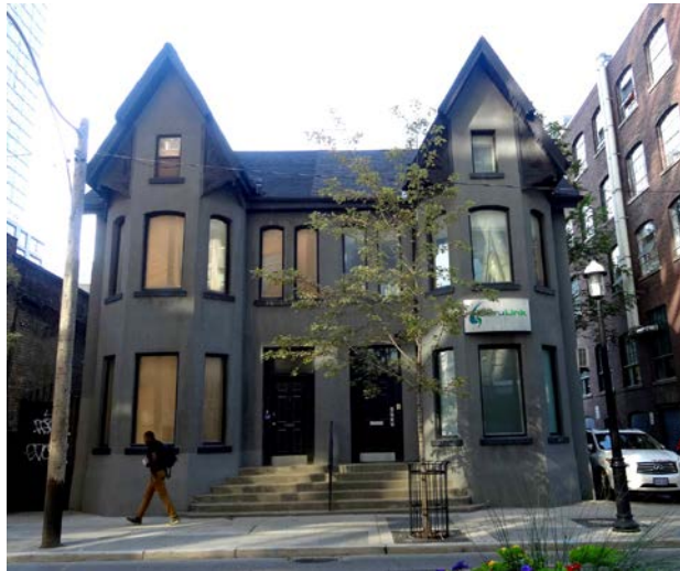
Current photograph, showing the principal (east) elevations of the properties at 357 and 359 Richmond Street West (Heritage Preservation Services, 2015)
