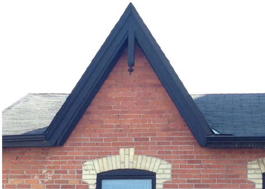
14. 813 Broadview Avenue : showing the turned finial in the gable ( Heritage Preservation Services, 2015 )
