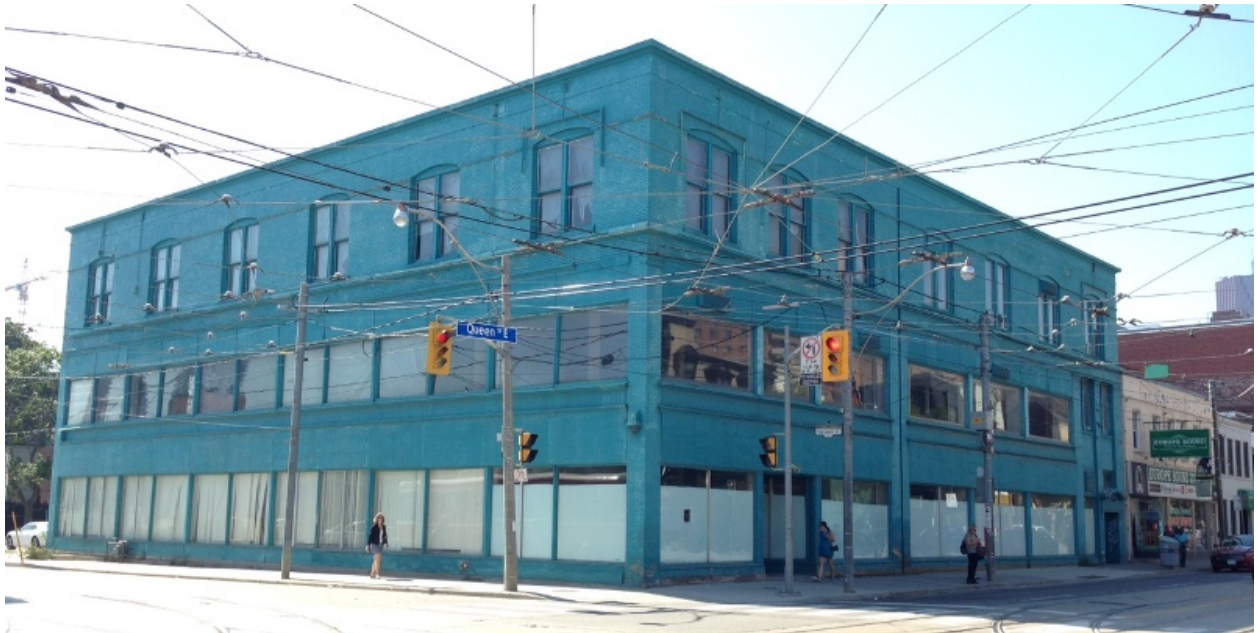
Showing the principal east and north façades of 339 Queen Street East Southwest corner of Queen Street East and Parliament Street (Heritage Preservation Services, 2015)
