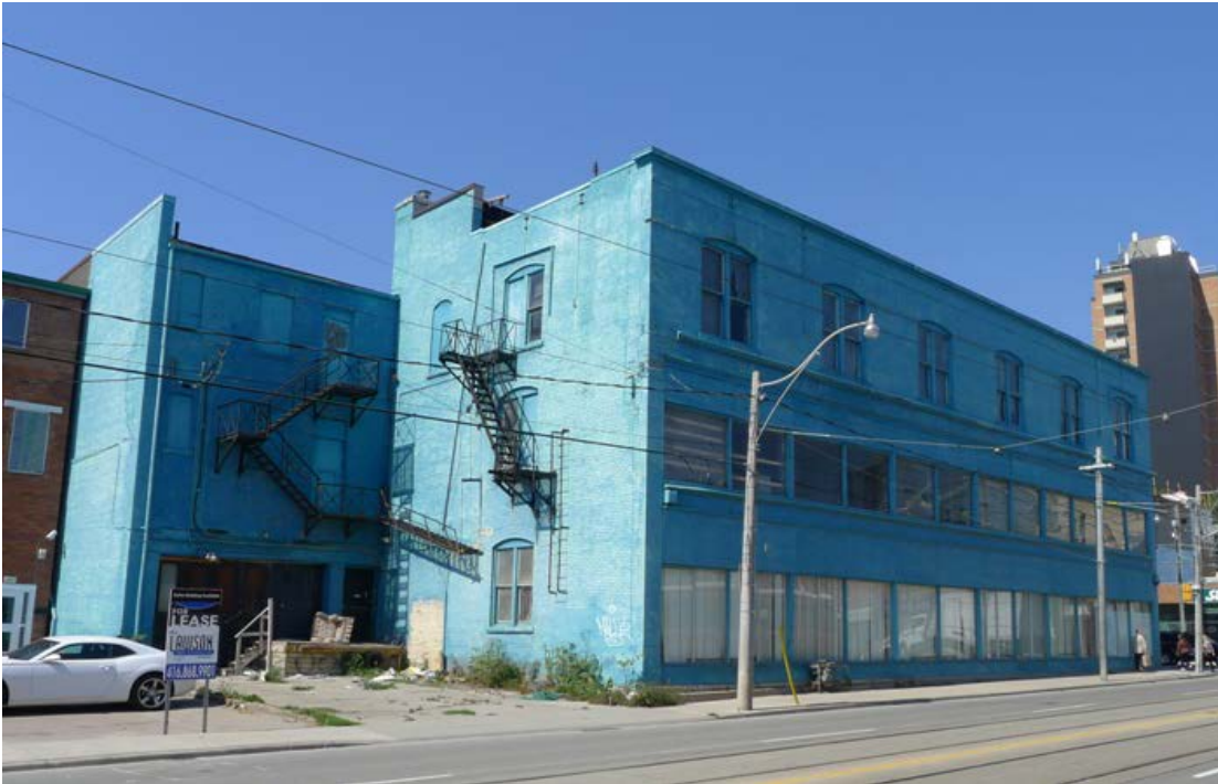
17. HFCC, south and east elevations facing Parliament Street : showing the east elevations with the window transoms covered over with boards and the south elevations indicating the extent of the original 1907 and the larger extension of 1925-6 (left of photo). (HPS 2015)
