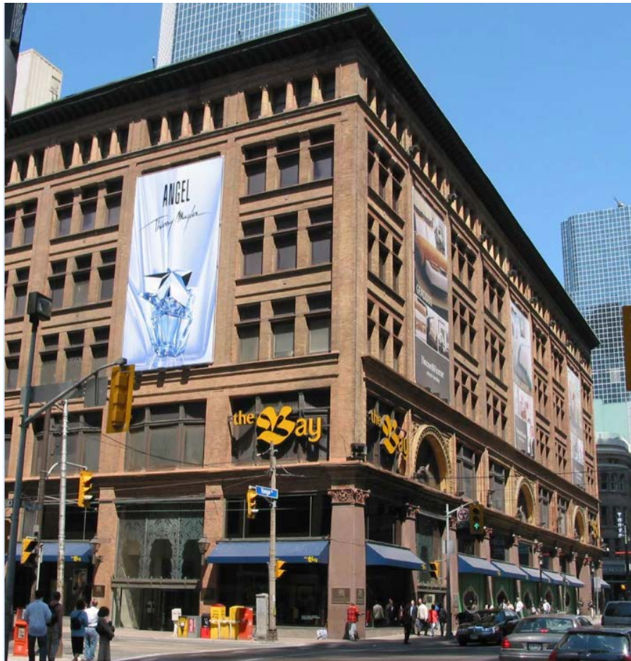
9. The Robert Simpson Company, 176 Yonge St, Edmund Burke (1894-5), Burke & Horwood (1899-1900), Horwood & White (1922-4): showing the large glazed openings at the first two floors, smaller windows at the upper floors, differentiated attic floor and overhanging cornice. A combination of granite with brick and decoratively relieved terracotta panels is employed for cladding. ( TOBuilt )
