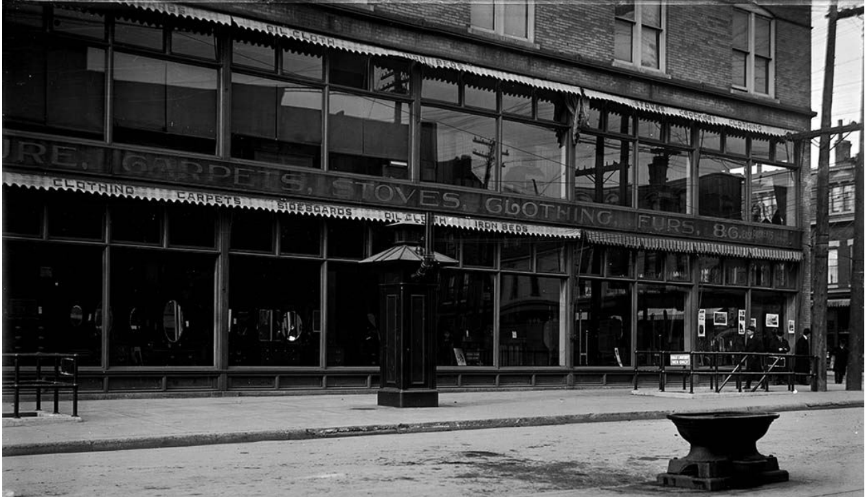
13. HFCC, east façade on Parliament Street , 1914 (detail) : showing the details of the glazing on the two lower floors, with the large glazing panels grouped in pairs between the minimal vertical structural supports with transom lights divided into pairs above each large pane, and the narrow paired panels at grade. At the third floor segmental arched windows contain a pair of double-hung sash. Note the brick entablature and moulding between the second and third floor and the narrow signage panel between the first and second floors. ( City of Toronto Archives, Fonds 1231, Item 1295 )
