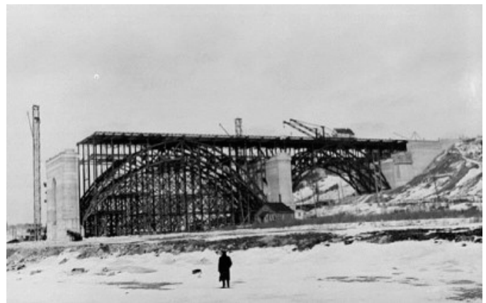
Construction of Prince Edward Viaduct c1915 (National Archives of Canada PA-070098).
