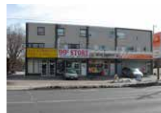
Bater's General Store site at 1129 Broadview Avenue, 2015
