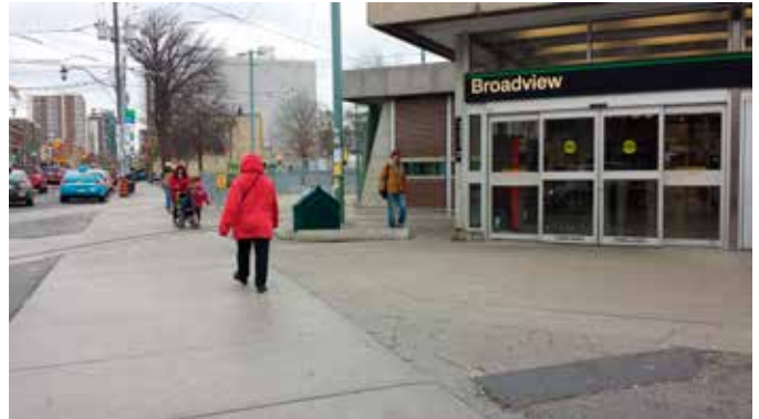
Broadview TTC subway station
