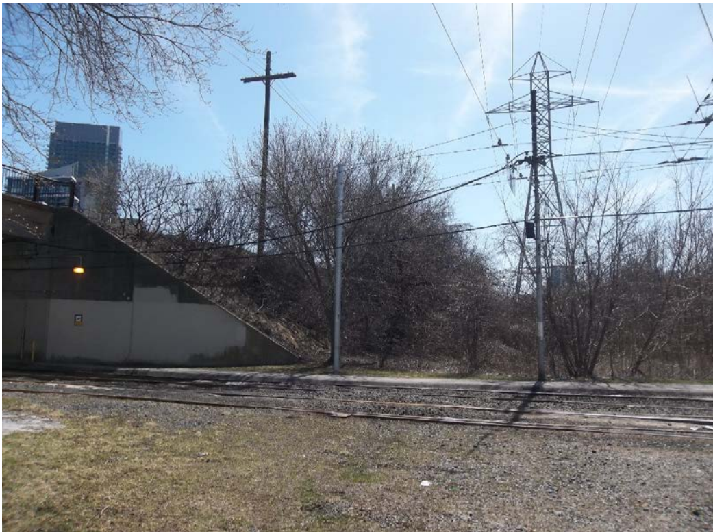
5) Humber Loop looking southwest to future GO Transit station/pedestrian tunnel location
