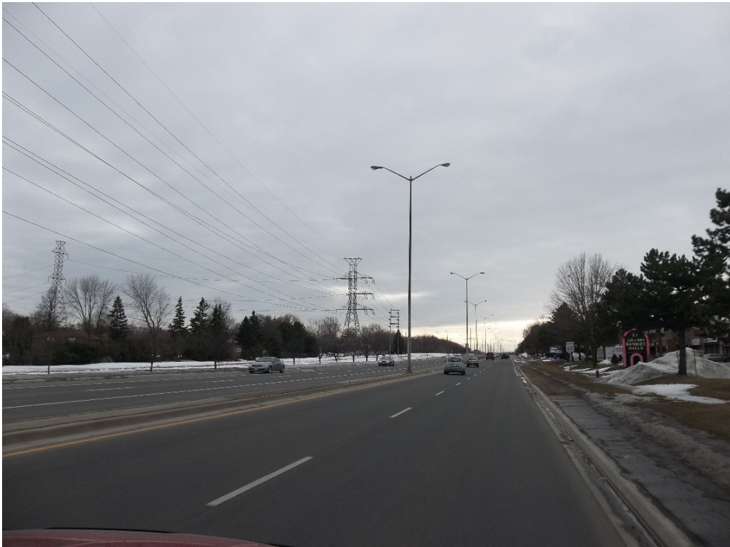
14) The Queensway, looking west from west of Dixie Rd.
