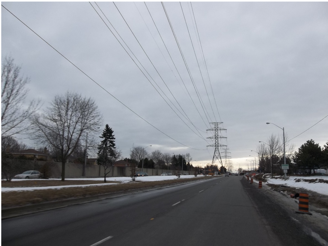
13) The Queensway (now widened), looking west from east of Dixie Rd.
