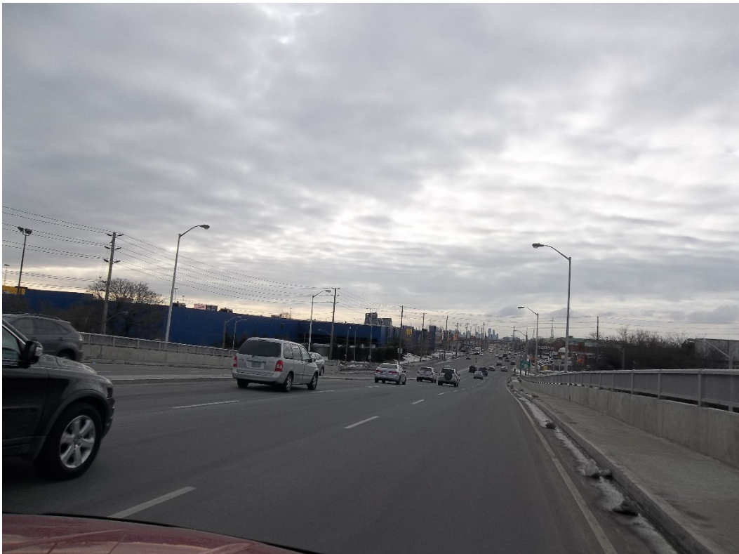
9) The Queensway, looking west from west of Kipling Ave.
