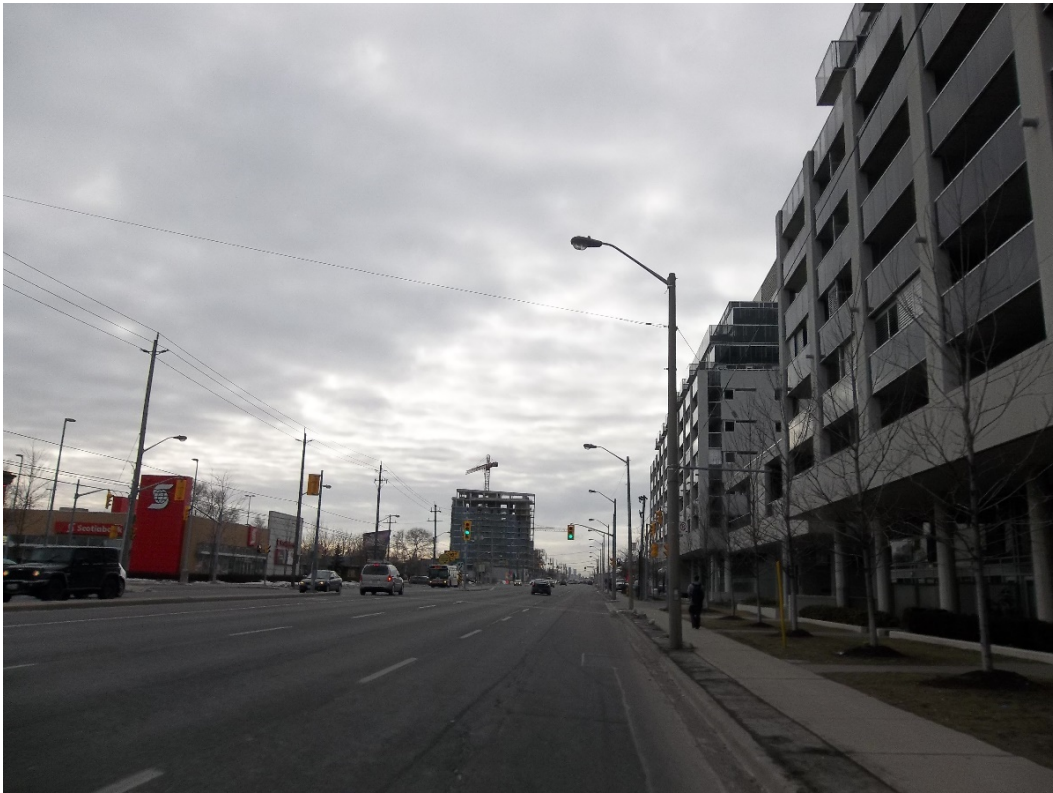
8) The Queensway, looking west from west of Islington Ave.
