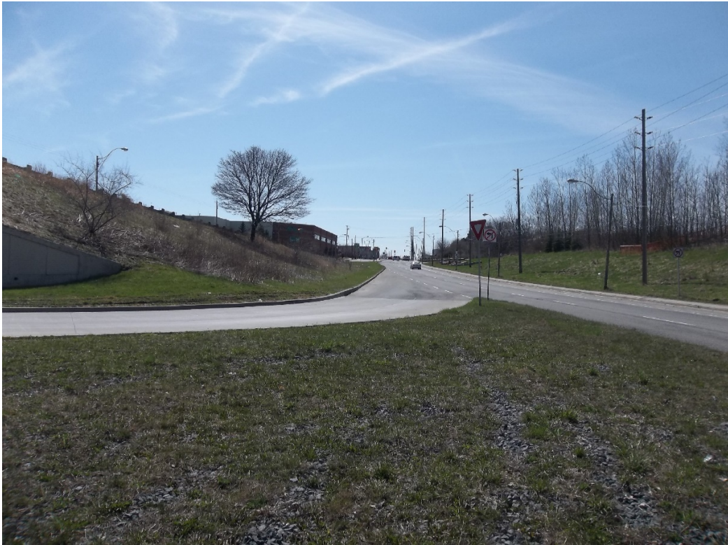
7) SEMALRT westbound route at Humber Loop exit to The Queensway, looking west (platform area)
