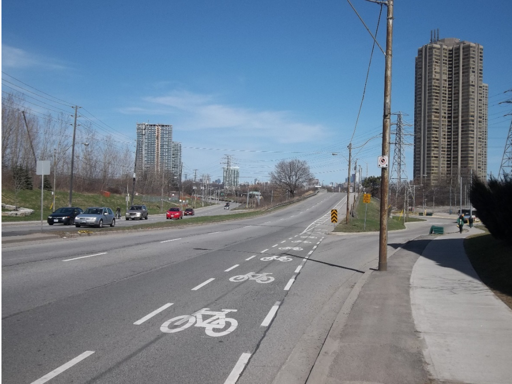
1) Eastbound approach from The Queensway to Humber Loop (at right)
