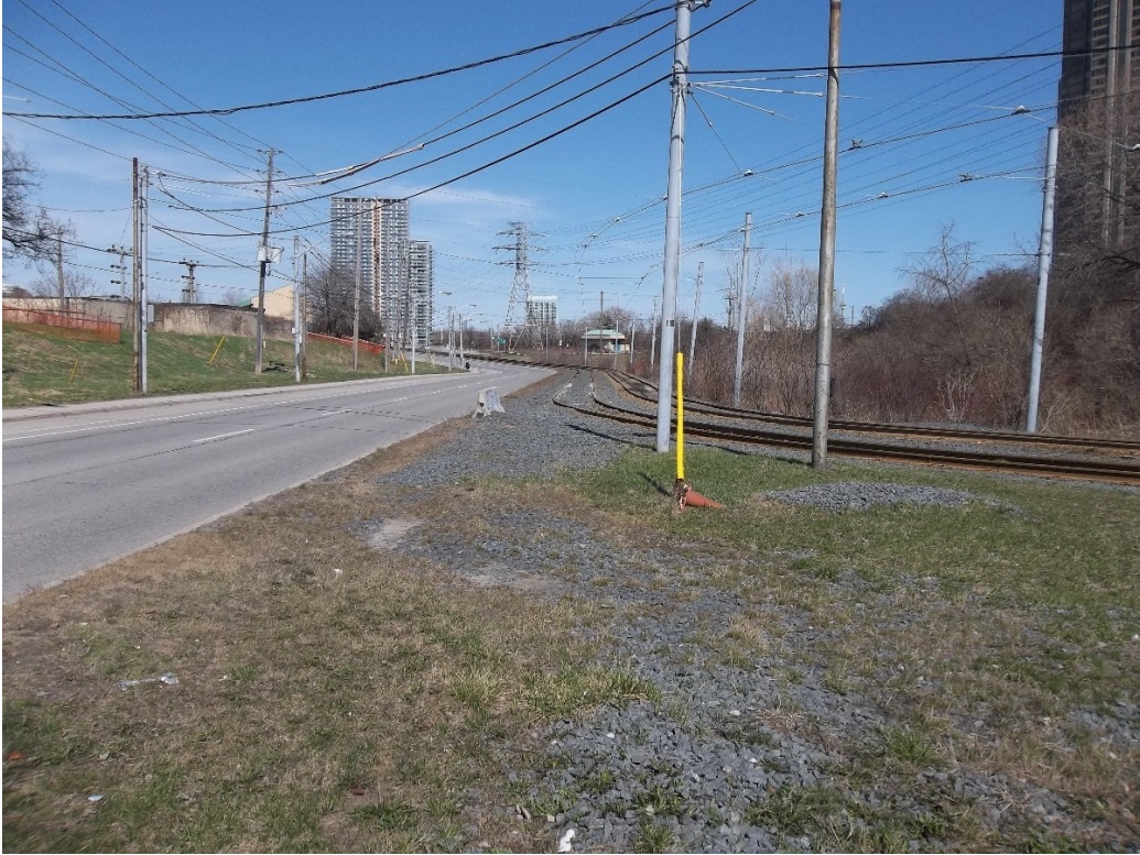
8) Sunnyside Streetcar Line route alignment looking east from Humber Loop area along TTC R-O-W
