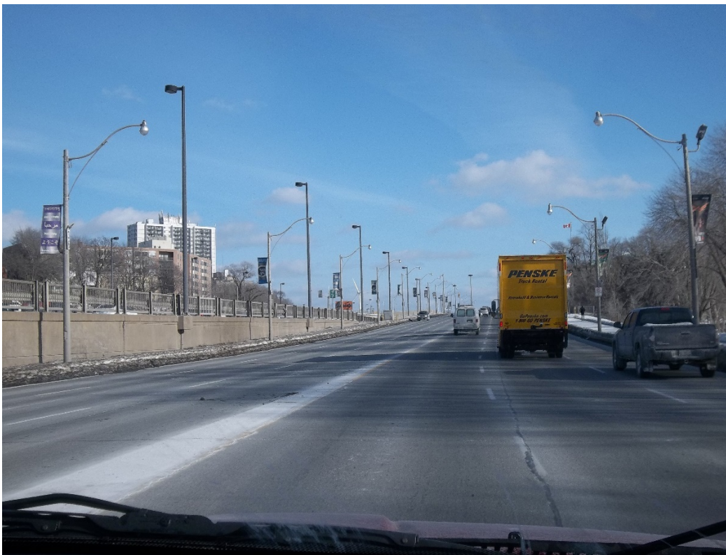
15) Median allowance termination, Sunnyside, looking east on hill
