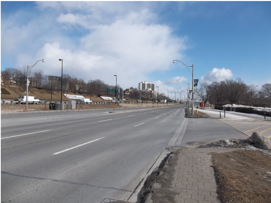
13) Narrow median allowance, Sunnyside, looking east at Boulevard Club
