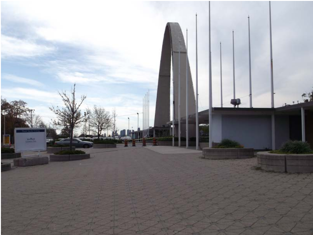
28) C.N.E. at Dufferin Gate, looking west along streetcar route
