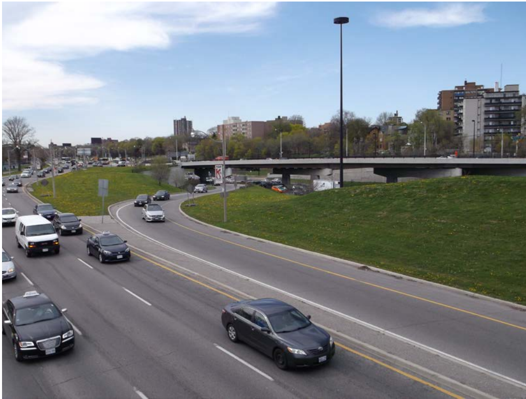
20) Lake Shore Blvd. West, streetcar bridge route looking west to tunnel exit (greenspace at left)
