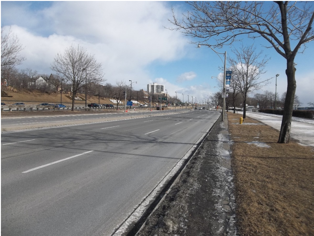
12) Narrow median allowance, Sunnyside, looking east from east of Palais Royale
