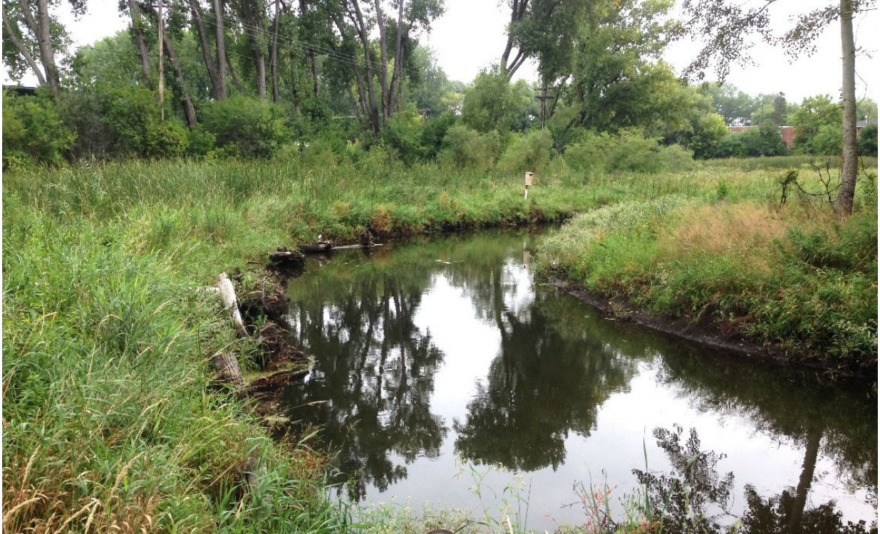
Figure 18 Example of Bioengineered Bank - soil at river's edge is encapsulated in biodegradable fabric to prevent erosion as plantings become established.
