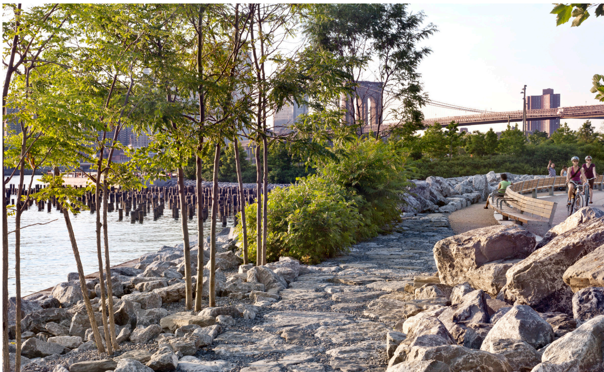
Figure 17a Example of Exposed Armour - boulders and large cobbles are used in critical areas to resist erosion from flood events and provide access to the river's edge.
