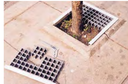
Optional protective tree grate being installed
