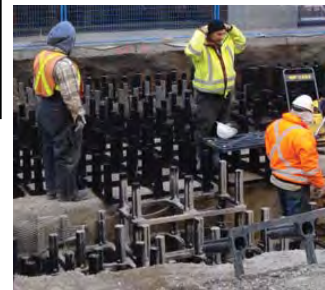
Example of soil cells being installed (Bloor St. W.)
