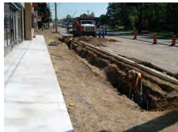
Continuous soil trench under construction
