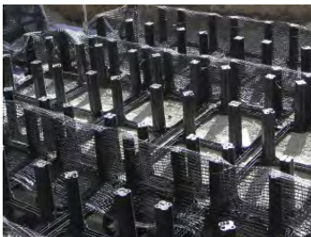
Structural soil cells during construction
