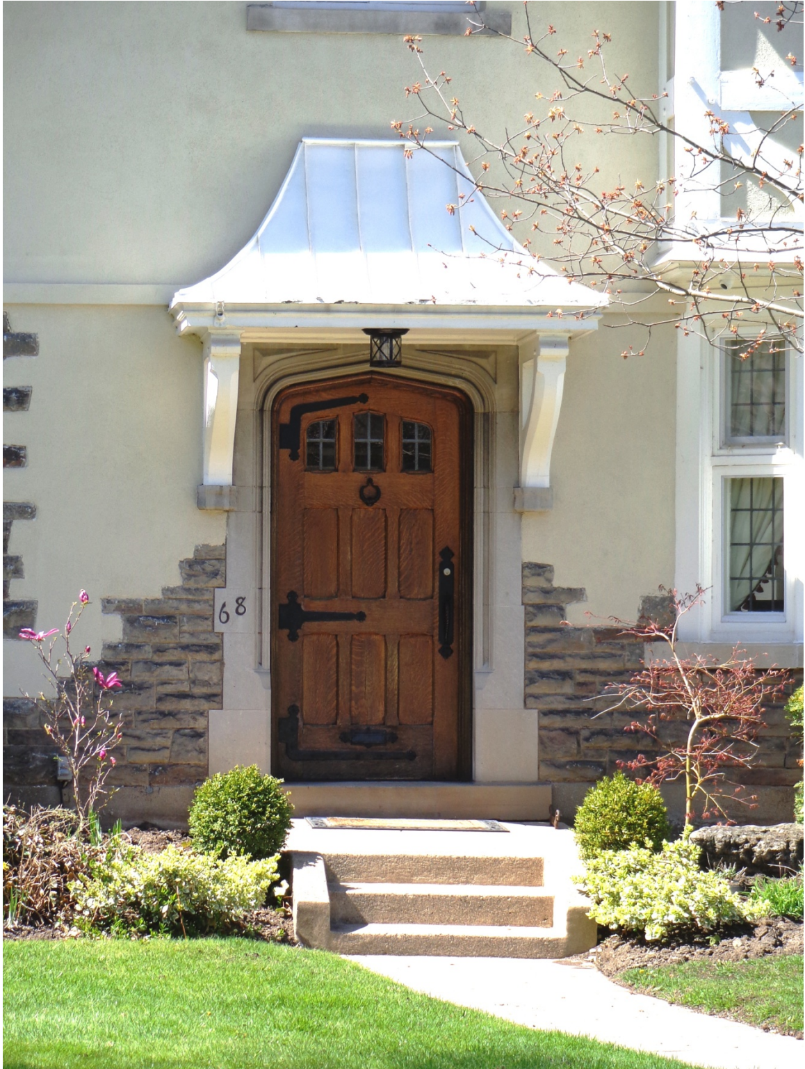
29. Front Entrance, South Elevation : showing the panelled wood door with the leaded lights, elaborate strap hinges and door handle with a moulded stone surround with a flattened pointed arch and adjacent rough-hewn river stone foundation ( Morgan, 2016 )
