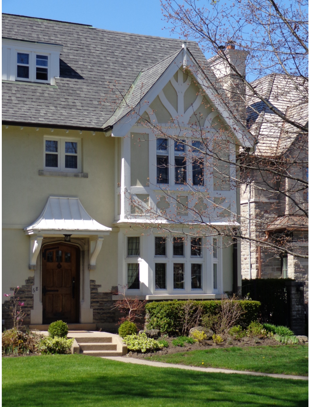
26. South Elevation, East Bay : showing the projecting octagonal ground floor bay window, with the second floor jetty with the half timbering and quatrefoil motifs and drop pendant in the apex of the gable ( Morgan, 2016 )
