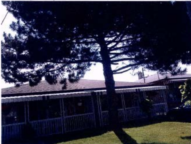
Picture 2. From north west, overview of lower canopy, note wire on left and hydro mast to #145 on right. Downspout at base of tree trunk in what is supposed to be a swale.
