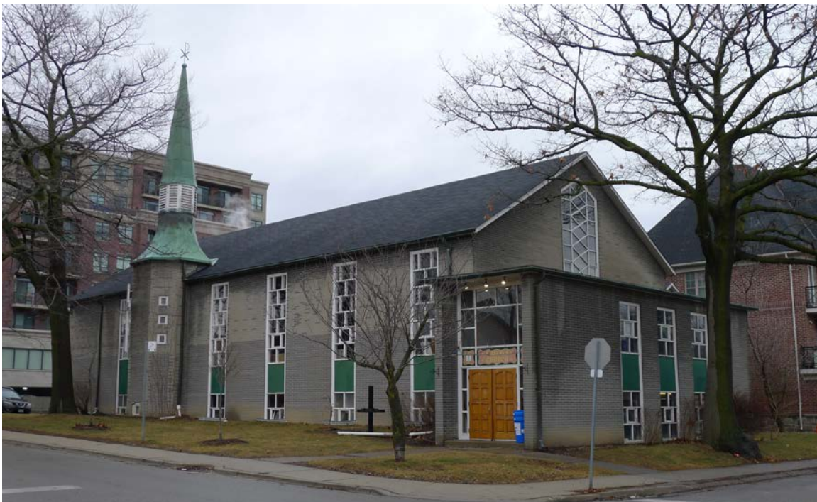
Showing the west and south elevations of former St. Agnes' Church, 69 Long Branch Avenue with the church, spire and narthex (entry) block. (Heritage Preservation Services 2016)
