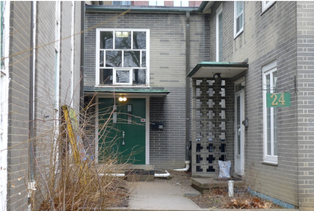
24. St. Agnes' Church, entry to rectory and chapel/office : showing the two minor entrances of the church complex with their projecting flat roof canopies. That of the rectory features a brick screen of pierced crosses. (HPS, 2016)
