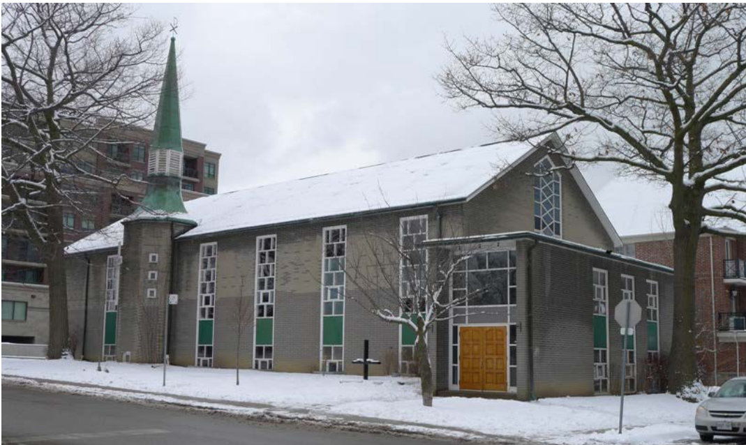
18. St. Agnes' Church, south and west elevations: showing the church, baptistery with steeple and entry narthex at the north-east corner of Long Branch Avenue and Marina Avenue. Note the later doors in the entry. (HPS, 17 February, 2016)
