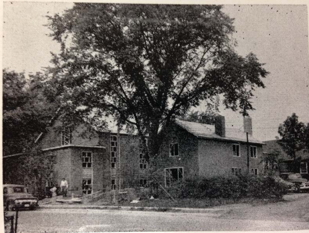
13. St. Agnes' Church, 69 Long Branch Avenue, during construction, c 1958 : showing a view from Marina Avenue of the new church (left) and new rectory (centre) with the remaining old church prior to demolition (far right) (AAD)
