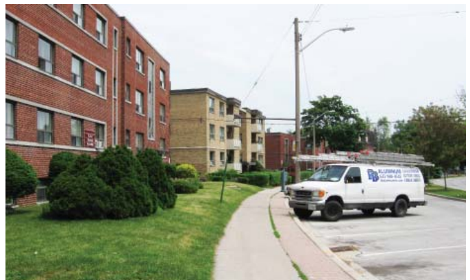
Figure 22: 8-12 Anglesey Boulevard Looking East
