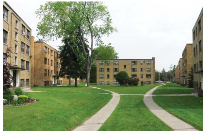
Figure 2: Looking East at 11 Bexhill Court
