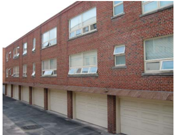
Figure 31: Rear of 24 Anglesey Boulevard
