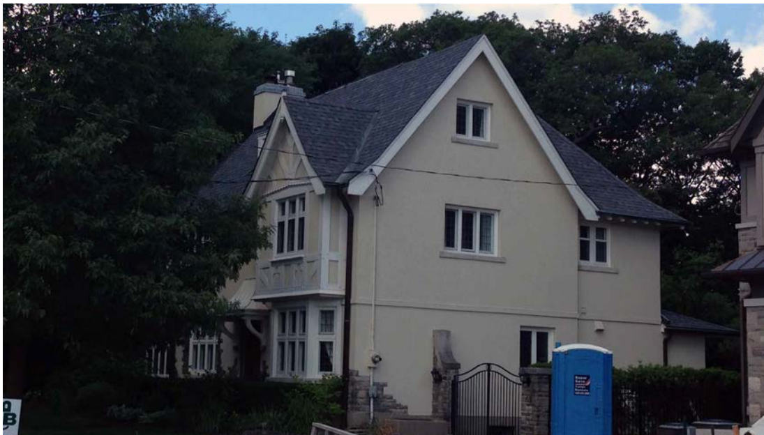
68 Baby Point Road: principal (south) elevation (above) and side (east) elevation (below)
