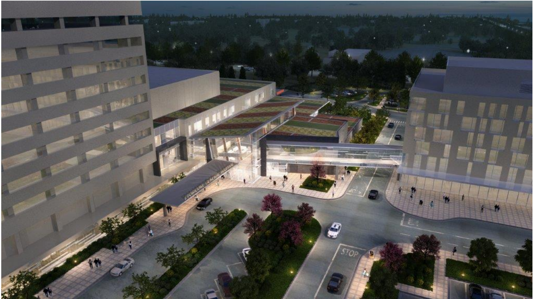
NPT (left), Bridge Connection, ASB (right)
