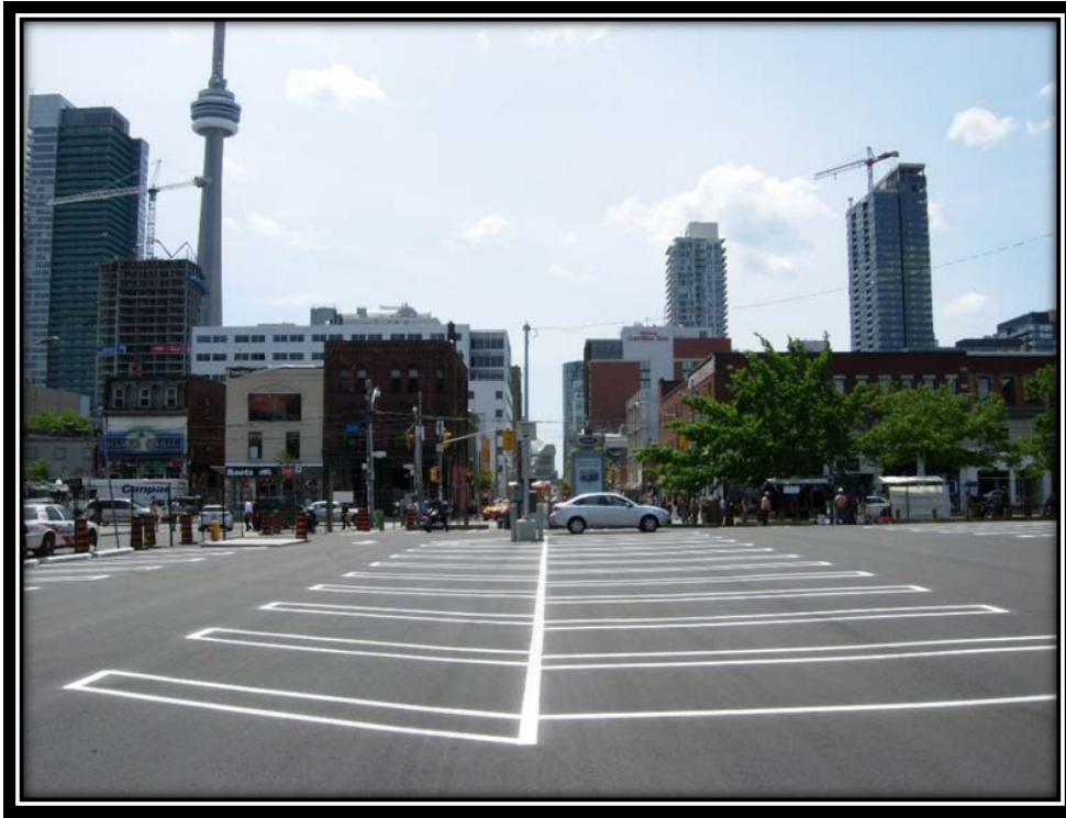
Municipal Carpark 262 (300-308 Queen Street West)
