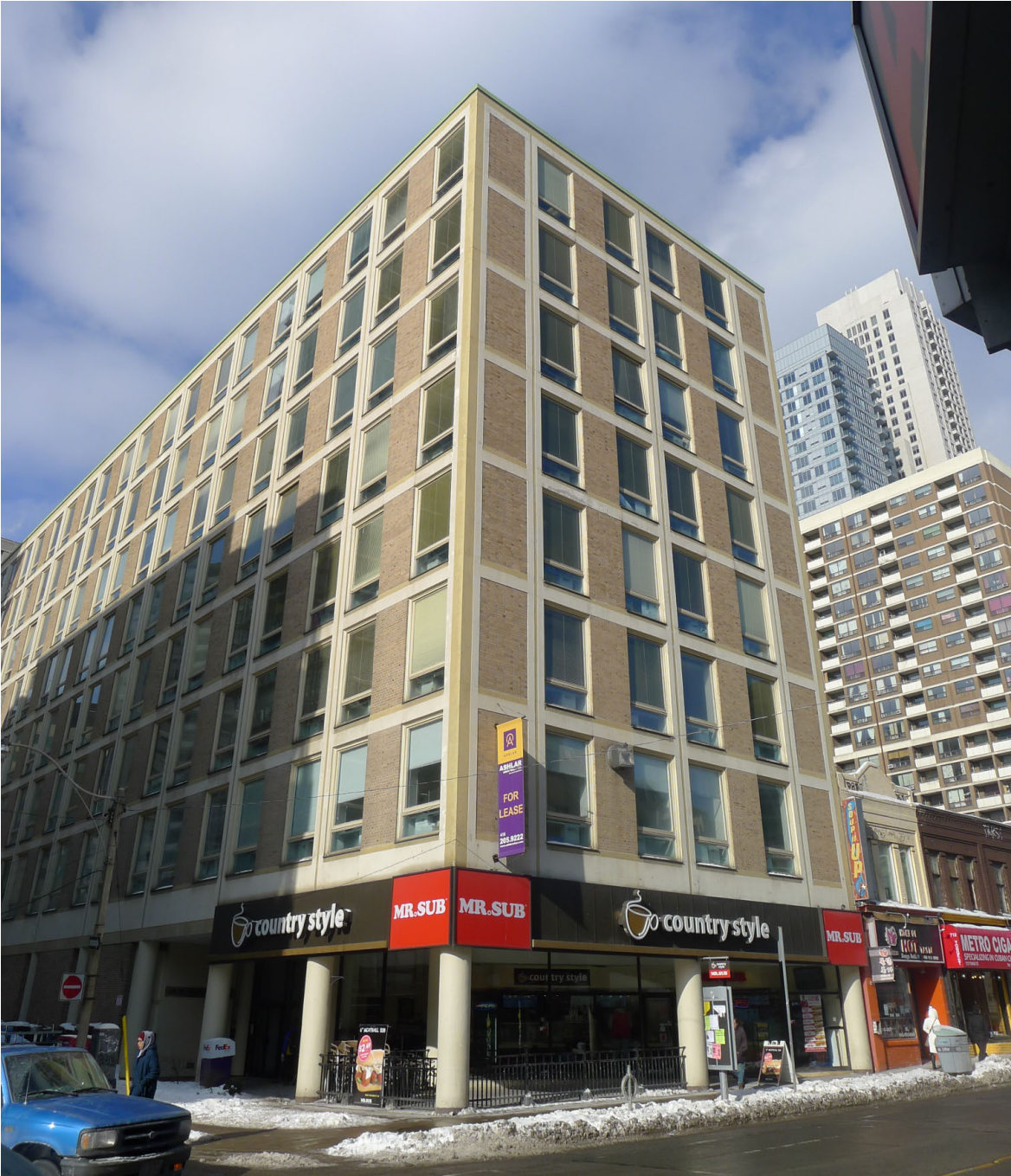
View looking north-west
