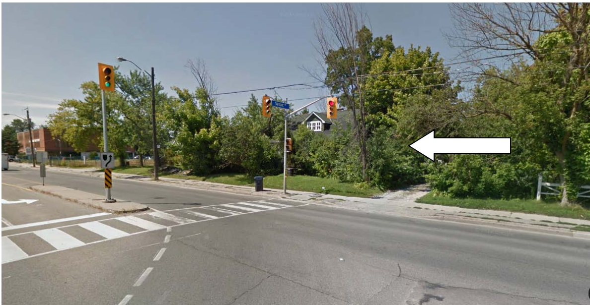
View of the Arthur Waine House, looking northwest on Finch Avenue West
