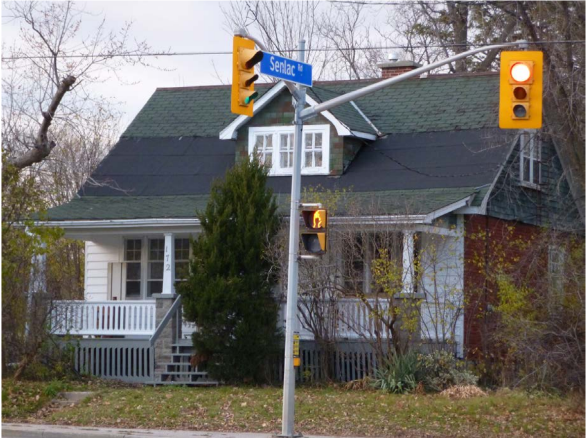
View of the Arthur Waine House from Finch Avenue West
