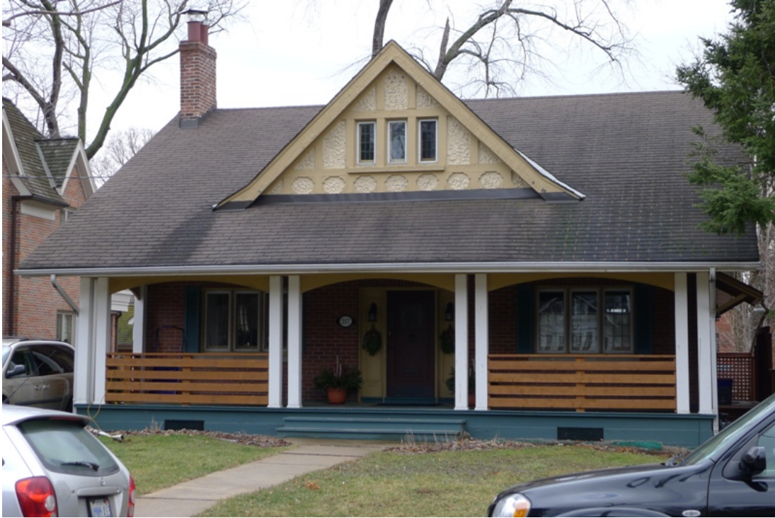
8. Forsey Page House, 217 Sheldrake Boulevard : showing the front (north) elevation with the broad gable roof, overhanging a deep porch with a gable dormer with Tudor half timbering and stucco. (HPS, 2016)
