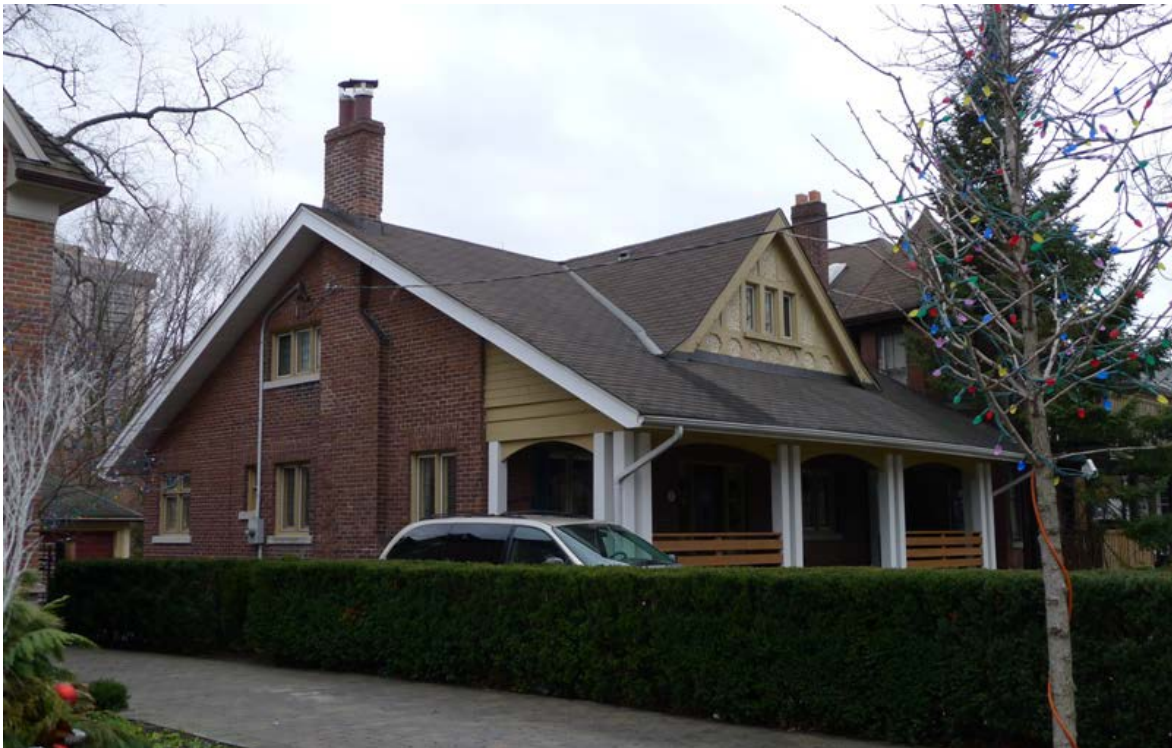
9. Page House, east and north elevations : showing the extent of the broad gable roof, depth of the verandah and east elevation with chimney. (HPS, 2016)
