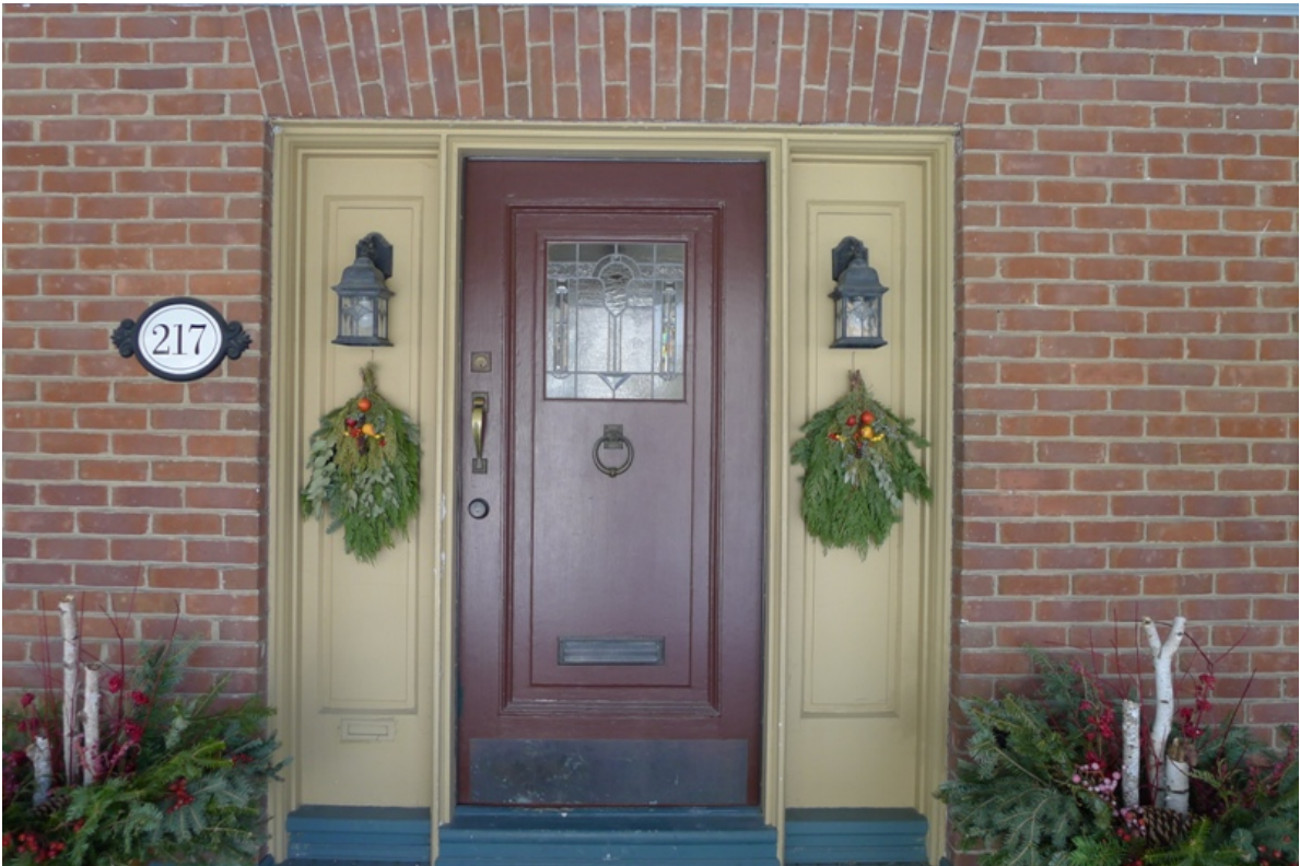
11. Page House, front door : showing the typical pattern of a central door framed by sidelights. (HPS, 2016)
