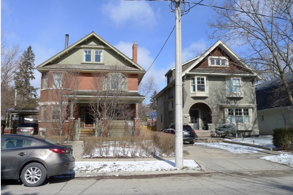
26. Sheldrake Boulevard, north side : showing the context with the variety of styles, materials and types, 124 and 128 Sheldrake. ( HPS, 2016 )
