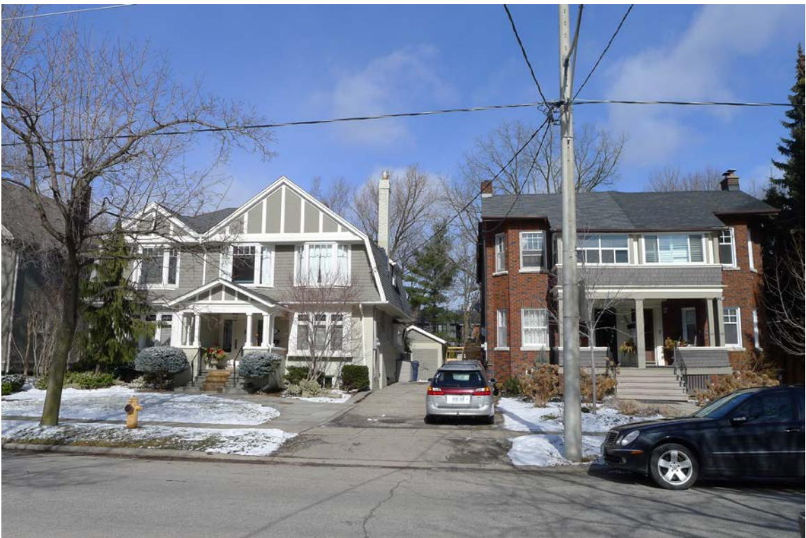
25. Sheldrake Boulevard, north side : showing the context with the variety of styles, materials and types, 136 Sheldrake (left) (HPS, 2016)
