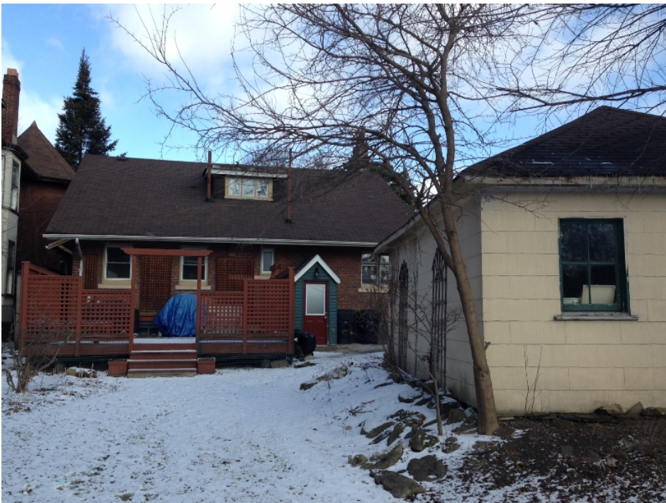
17. Page House, garage : showing the relationship of the garage to the house. (HPS, 2016)
