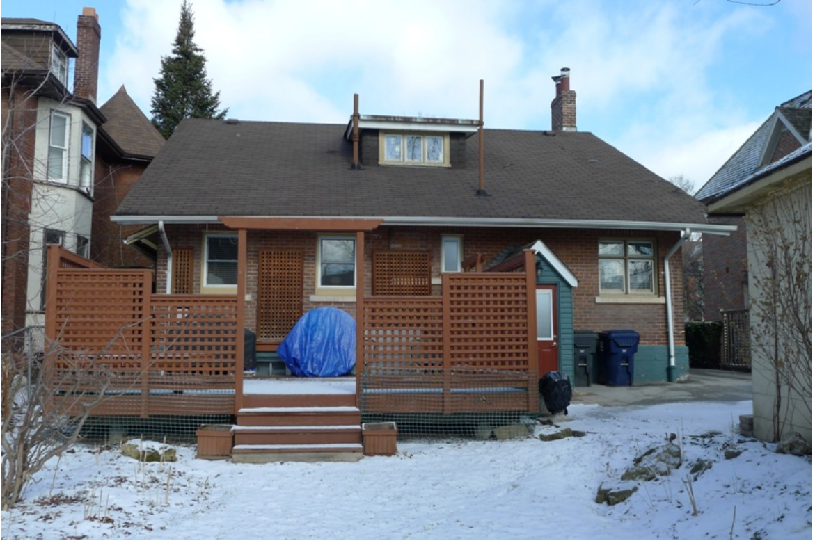
14. Page House, rear (south) elevation. (HPS, 2016)
