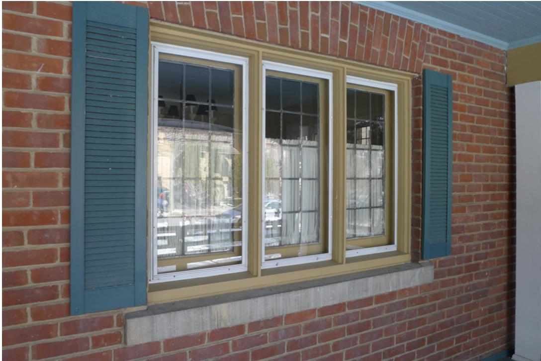
12. Page House, north elevation : showing a front window with its triple ligh, leaded glass and cast stone sill. (HPS, 2016)
