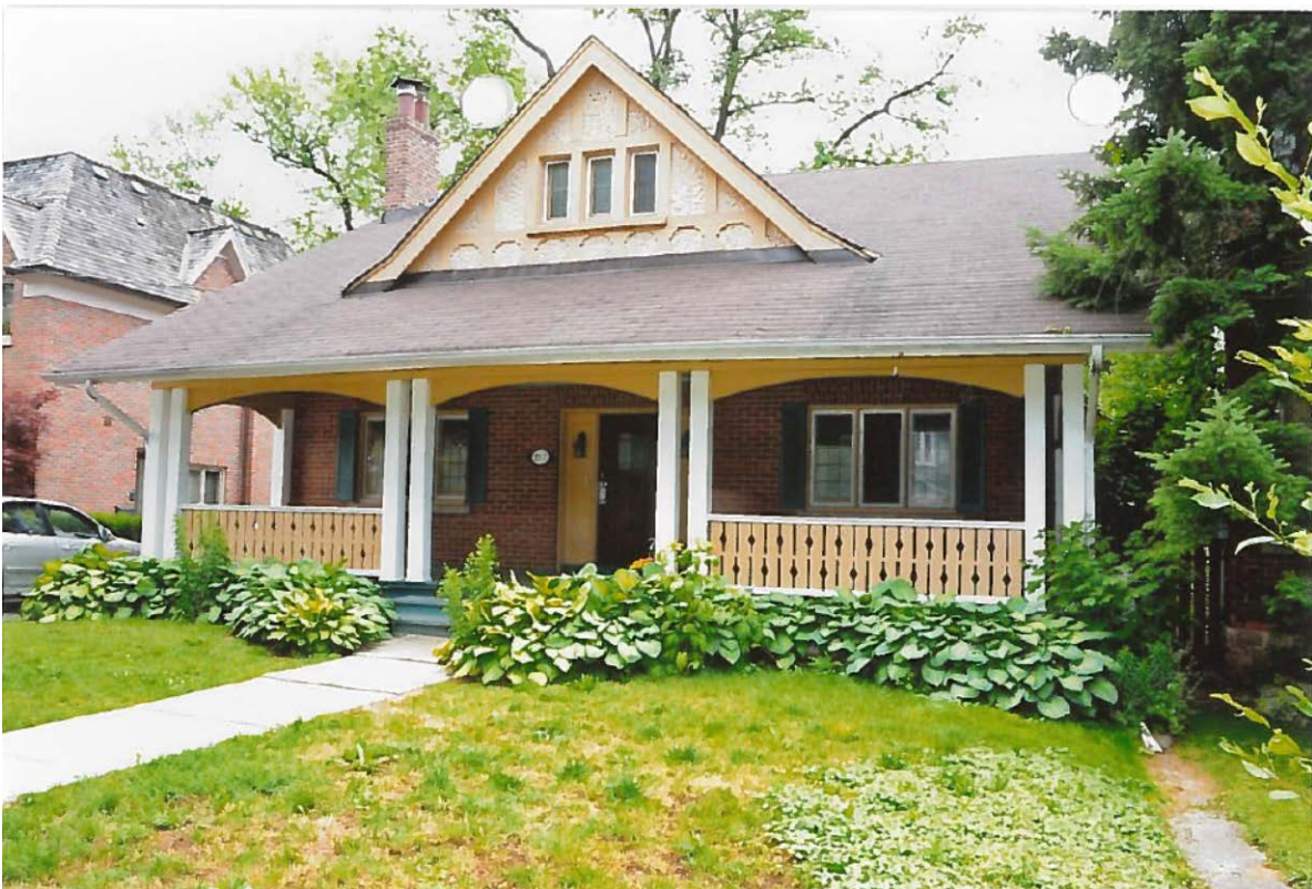
13. Page House, north elevation : showing the verandah with previous balustrade.(HPS files, 2012)
