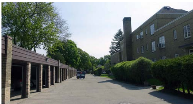
At the north end of the property, the garages are shown on the left, as well as the rear (north) wall of Building C with the three-part building and the large chimney.
