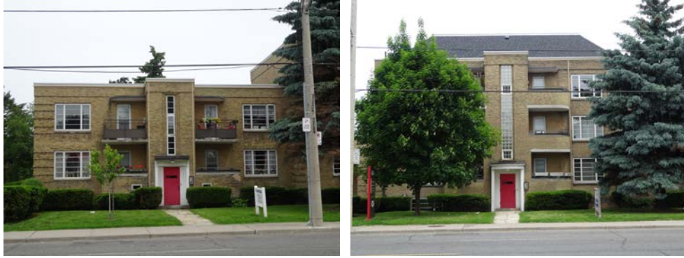
The west elevation of Building A on Bayview Avenue, showing the three-storey centre section (right) flanked by the two-storey north wing (left). Similar features are found on Building K on Bayview, Buildings E and F on Berney Crescent, and Buildings C and H facing the interior courtyard.
