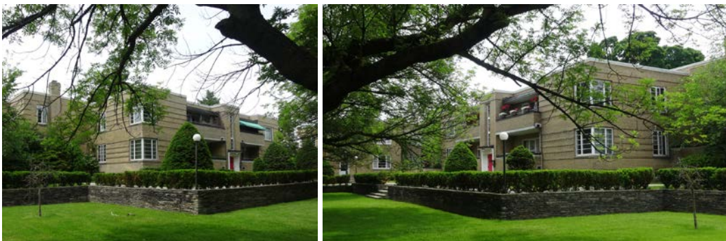
Showing Buildings B (left) and J (right), which anchor the northwest and southwest corners of the central courtyard, respectively (similar two-storey Buildings D and G anchor the other corners).
