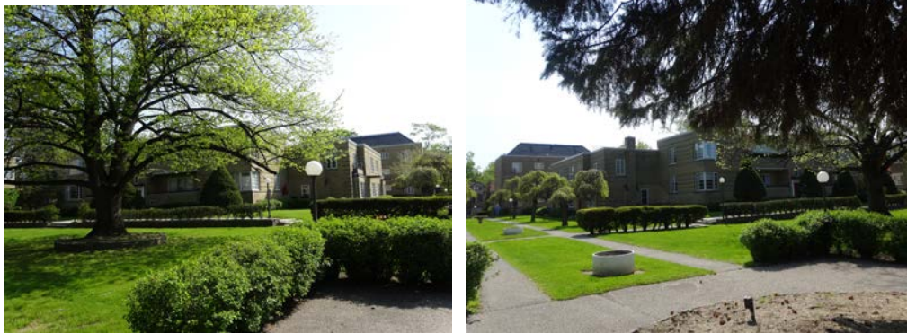
Looking east from the central courtyard and showing Buildings D (left) and G (right), which anchor the northeast and southeast corners, respectively.
