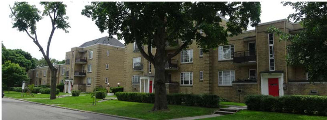
The west elevations of Buildings F (left) and E (right) on Berney Crescent, which forms the east boundary of the site.
