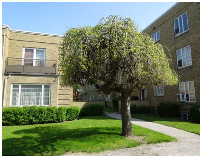
Showing the pathways and retaining walls between the buildings, in this case Buildings D and E.
