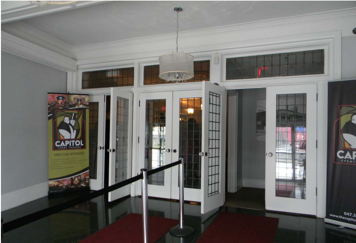
Showing the entrance lobby with three sets of doors with the multi-paned inserts and the flat-headed multi-paned transoms (Heritage Preservation Services, September 2016)
