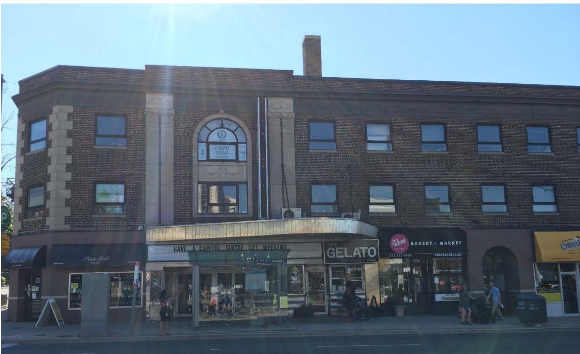
Showing the entrance to the Capitol Event Theatre. (Heritage Preservation Services, 2016)
