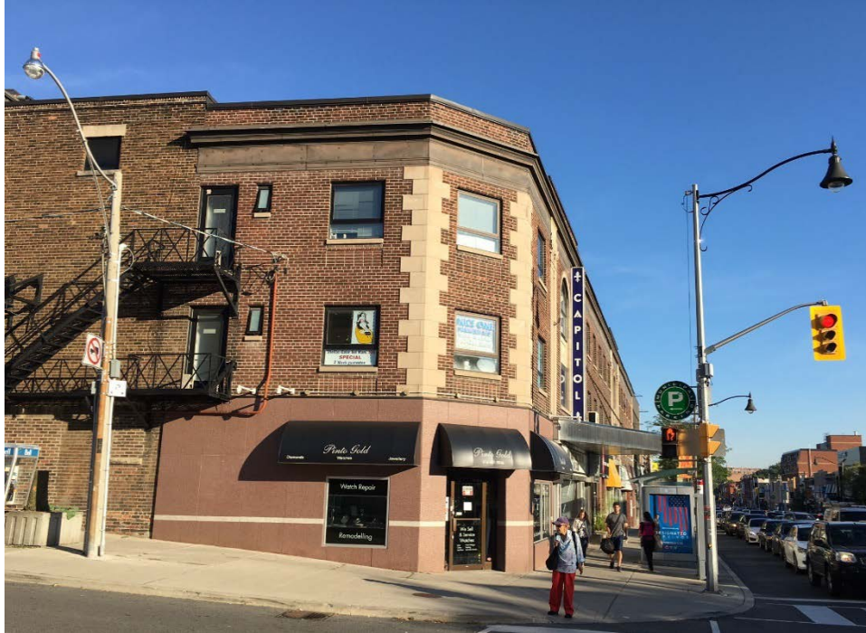
19. Current Photograph, 2490 and 2506 Yonge Street, 2016: showing the three storey complex, east of the York Theatre auditorium at the corner of Castledfield Avenue (above). Please note the different color of bricks. (Heritage Preservation Services).
