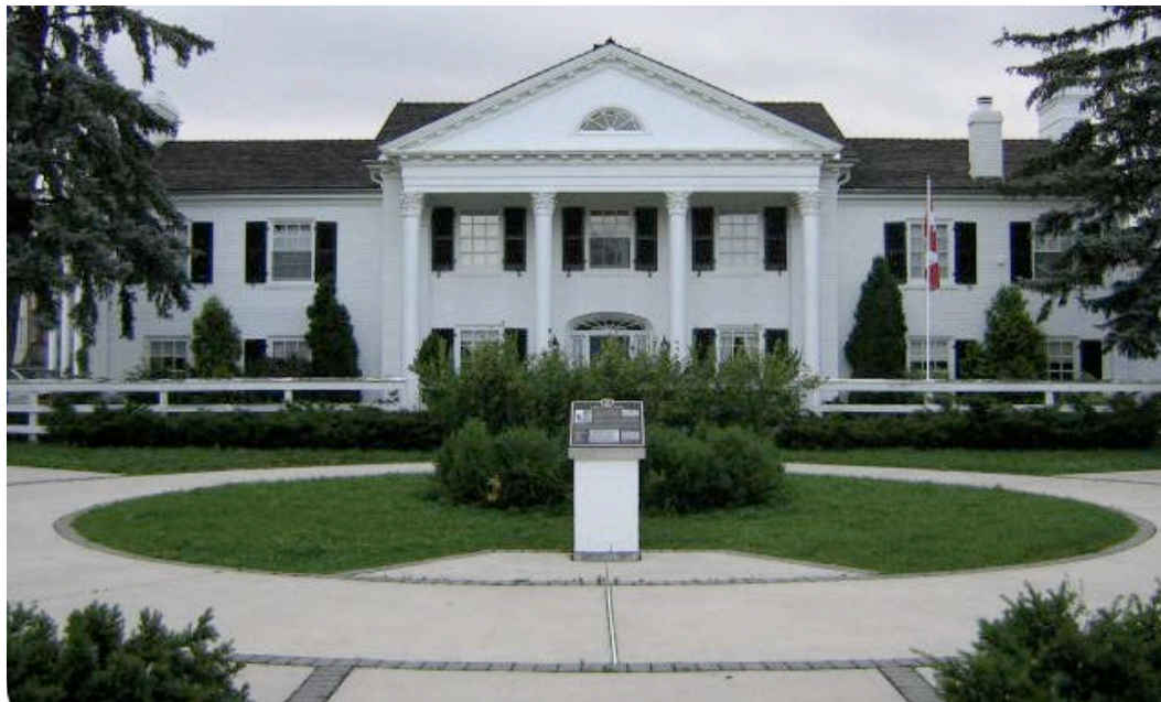
11. Photograph, Green Meadows Estate, undated: showing the estate house built in the 1940s for entrepreneur J. A. “Bud” McDougald, a business associate and the brother-in-law of Colonel W. Eric Phillips, which shared the painted white brick, low roofline, and classical detailing of the subject property ( http://torontoplaques.com/Pages/Green_Meadows.html ).
