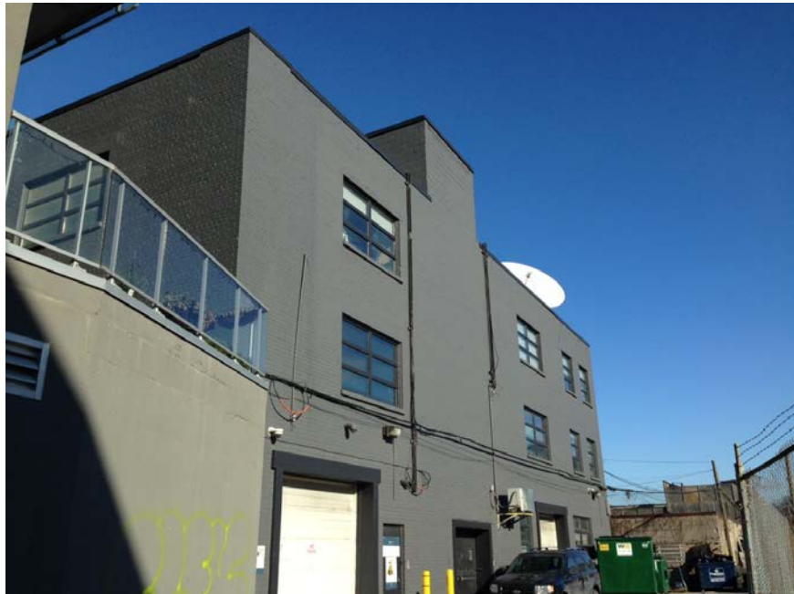
Showing the principal (north) elevation of 635 Queen Street East (top) and the rear (south) elevation (bottom) ( Heritage Preservation Services, 2016 )
