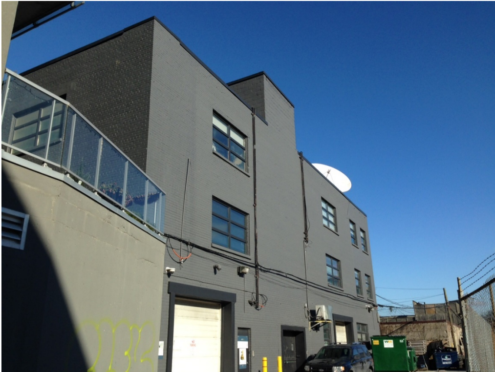
6. 635 Queen Street East : showing the rear, south, elevation. (HPS)
