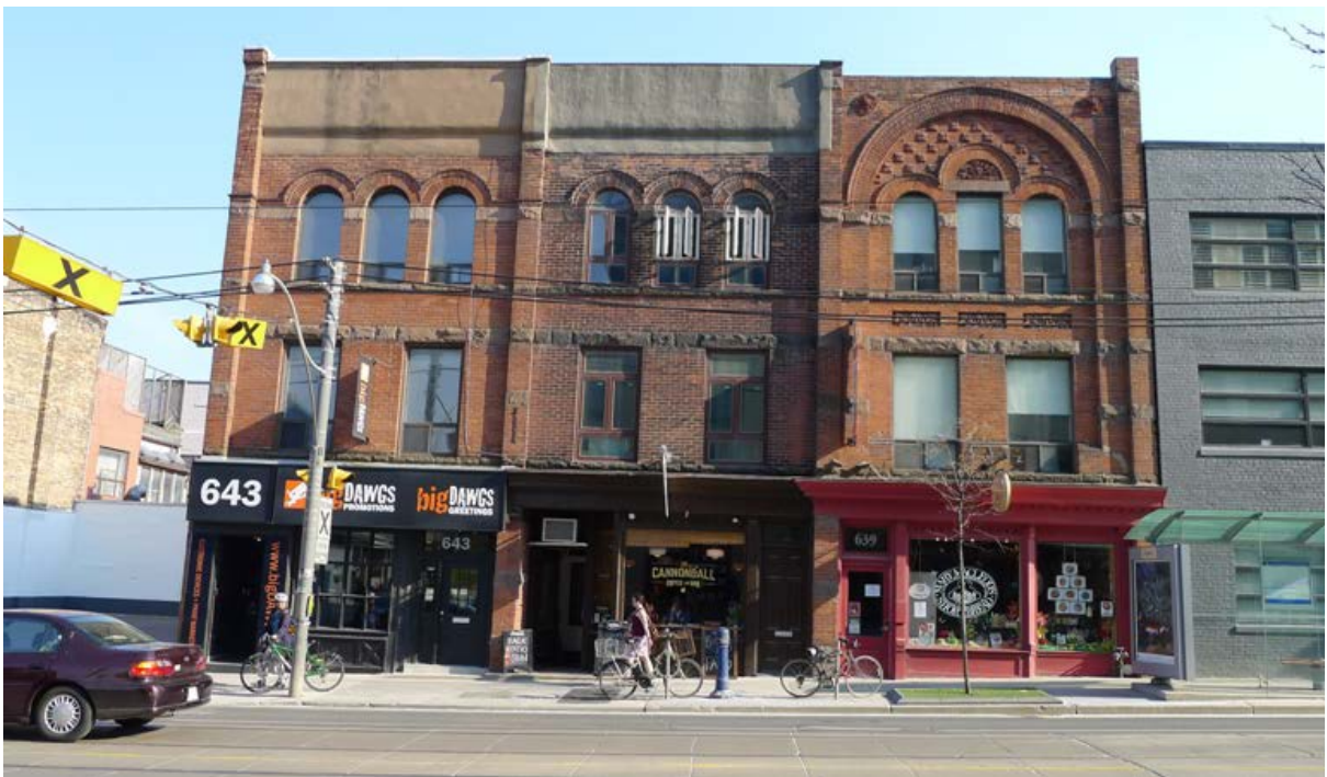
Showing the north elevations of the Smith Block properties at 639-643 Queen St. E. (HPS, 2015)
