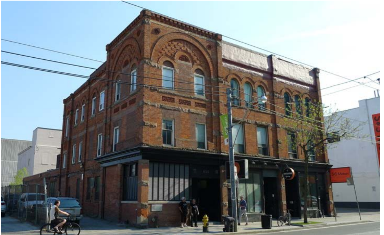
Showing the north and east elevations of the Smith Block properties at 651-655 Queen St. E. (HPS, 2015)
