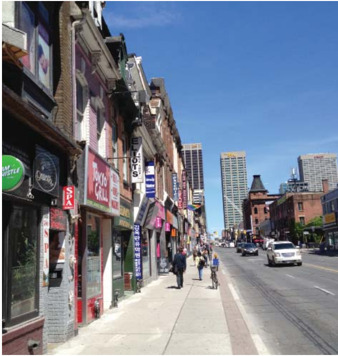
Example of mixed-use and commercial landscape along Yonge Street, looking north towards Gloucester Street, photo taken in 2013.
