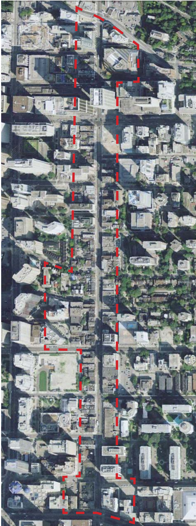
Aerial image from September 2009, illustrates changes in built form compared to figure 70. Study area (in red) is approximate.
