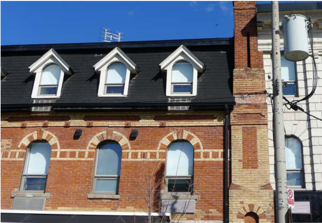
13. 1150 Queen Street West, west elevation, detail : showing the brick patterning around the windows, under the eaves and on the chimney. (HPS, 2016)
