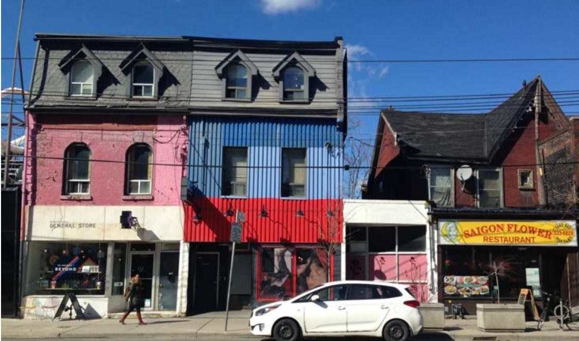
10. 1142 and 1144 Queen Street West : showing the two properties with the original design of the elevations with the pattern of shop front and two entrances at ground level, two semi-circular headed window openings at the second level and two gable dormer windows in the slate patterning of the mansard roof. Note the properties on the right, 1138 and 1136 Queen Street West, which contain the remains of a rough-cast, semi-detached house constructed in 1881. The white store at 1140 occupies what was originally the laneway of an earlier house. (HPS, 2016)
