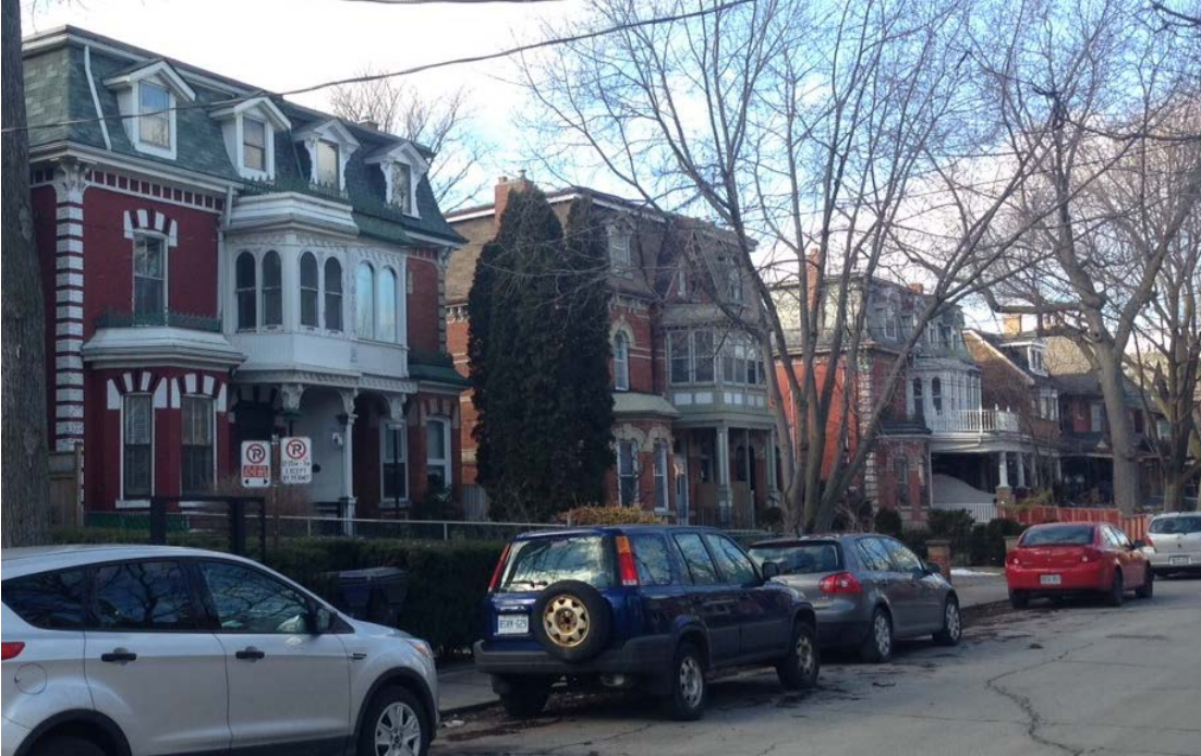
22. 28-30, 32-34, 38-40, Beaconsfield Avenue, west side : showing the context with the consistent two-and-a-half storey mansard-roofed houses with red and buff brick pattering including quoins, striped semi-circular window heads, quoins and a decorative band beneath the eaves. (HPS, 2016)
