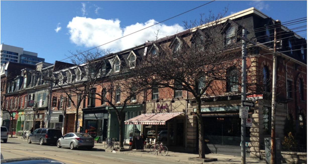
16. 1154- 64 Queen Street West : showing the block on the west side of Beaconsfield Avenue which corresponds in design and detail to that of the block on the east side at 1142-50 with the Drake Hotel. Note the consistency of height and /or use of mansard roofs in the blocks beyond 1164 Queen Street West ( HPS, 2016 )
