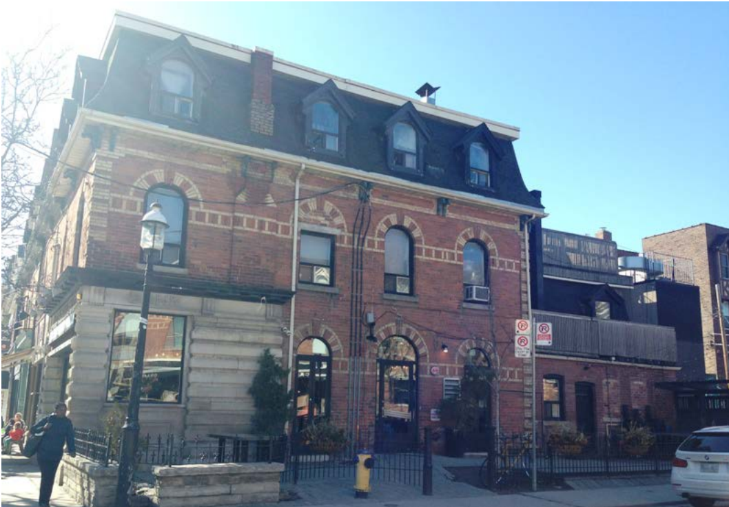
19. 1154 Queen Street West : showing the east elevation with the red and buff brick cladding patterns including the details around the windows and under the eaves as well as the dormer windows all of which match those at the Drake Hotel on the opposite side of Beaconsfield Avenue (Compare Images 12 and 13, above) ( HPS, 2016 )
