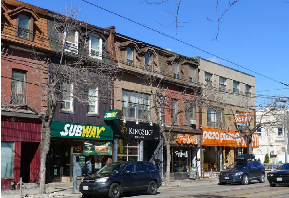
26. 1124-32 Queen Street West : showing the block west of the subject properties to Lisgar Street with the consistent two-and-a-half-storey height with mansard roofs, paired dormers and typically paired second floor windows. Note the quoins and bracket details which also survive. Note that the Pizza Pizza building conceals the mansard roof which is evident at the side elevation. (HPS, 2016)
