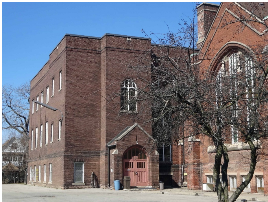
21. Current Photographs, Sunday School Building, 2016 : showing the east and west elevations (above) and the south and east elevations (below) with the east entrance (Heritage Preservation Services).
