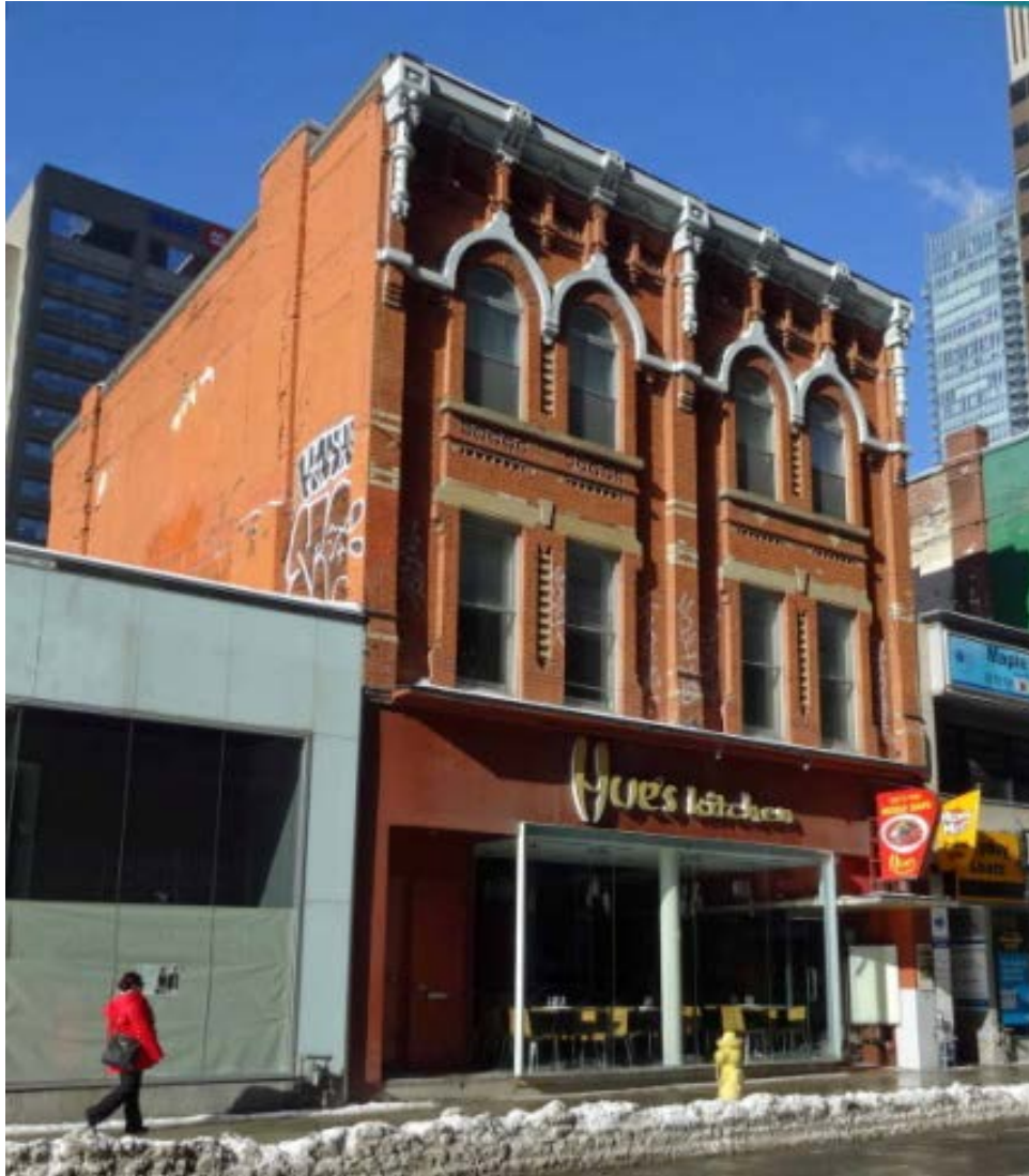
William Luke Buildings (1884) East Elevation View
