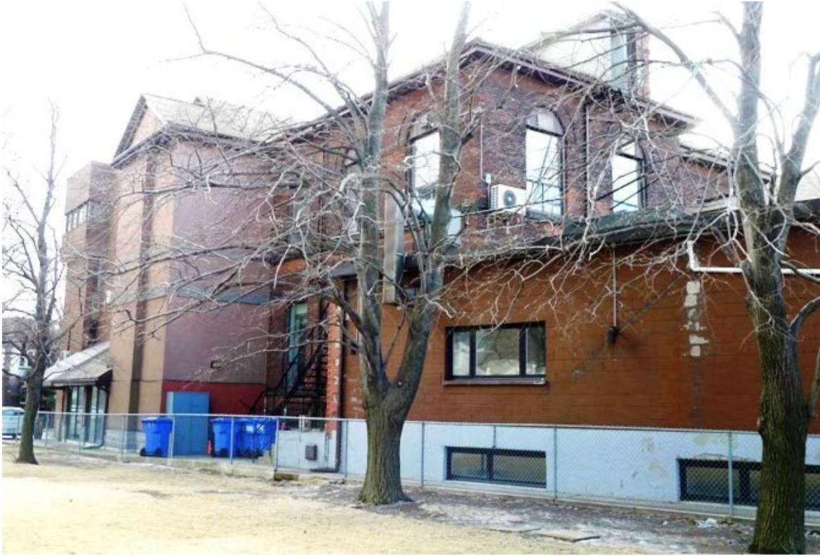
Above, photograph showing the north and west elevations with the 1975 addition at the far left, the 1995 entry and elevator tower addition (left) with the original school building in the centre and the 1962-3 addition with a single storey and a raised basement (right) (HPS)
