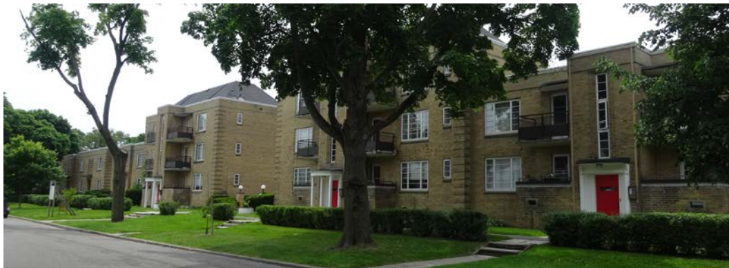
The west elevations of Buildings F (left) and E (right) on Berney Crescent, which forms the east boundary of the site.
