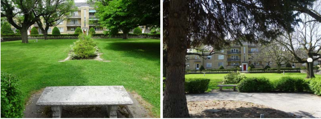
Buildings C (left) and H (right) face the central courtyard from the north and south, respectively.
