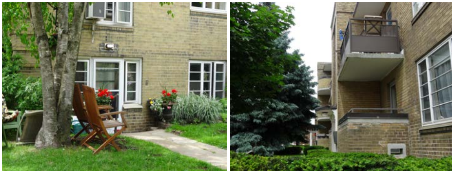
East (rear) elevation of Building A (left), and part of the west elevation of Building K on Bayview Avenue (right).
