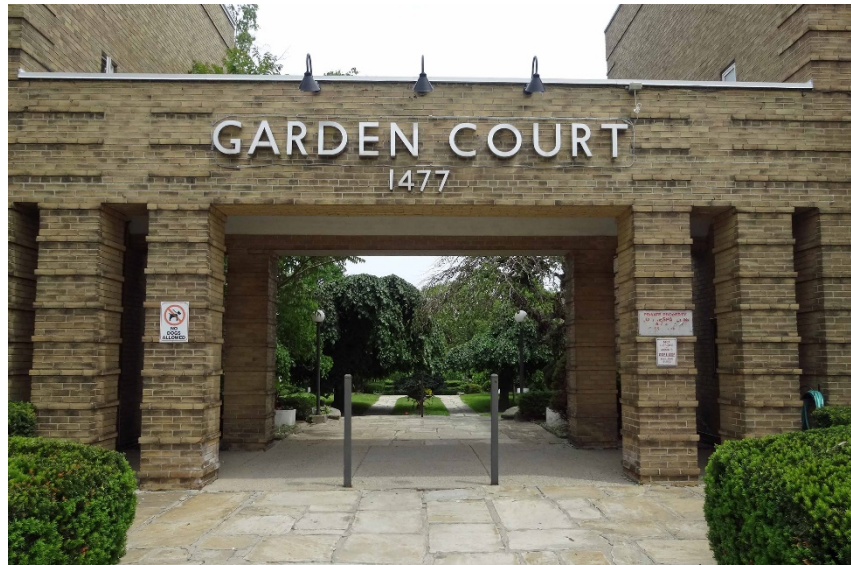
Above: the entrance to the Garden Court Apartments on Bayview Avenue; cover: the Bayview Avenue frontage, showing Building A (left) and Building K (right) (Heritage Preservation Services, 2016)
