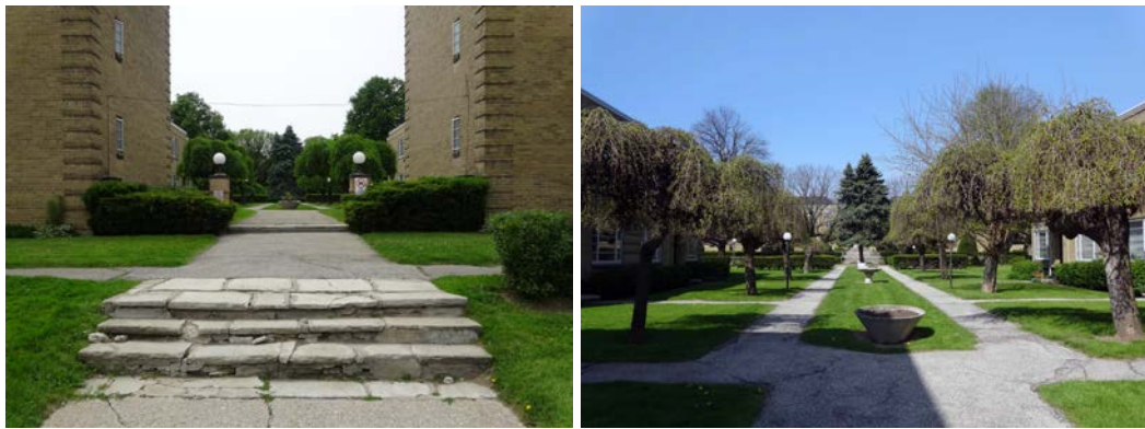
Views west from Berney Crescent between Buildings F and E with the lamp standards (left), and past Buildings G and D (right) to the central courtyard.
