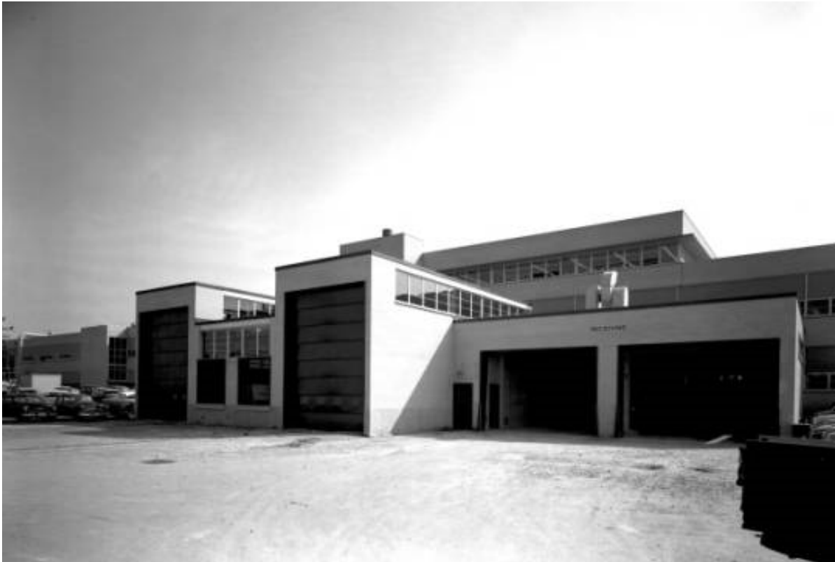
32. IBM Building West Elevation : showing the loading bays and offices above. (CAA, Panda,54416-2)
