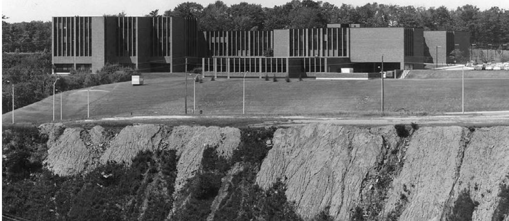
Above: 1150 Don Mills Road, IBM Headquarters Building, 1967 and 1971 looking north to the south and east elevations ( Panda Associates, IBMhq-07, NORR Architects, Engineers and Planners )
