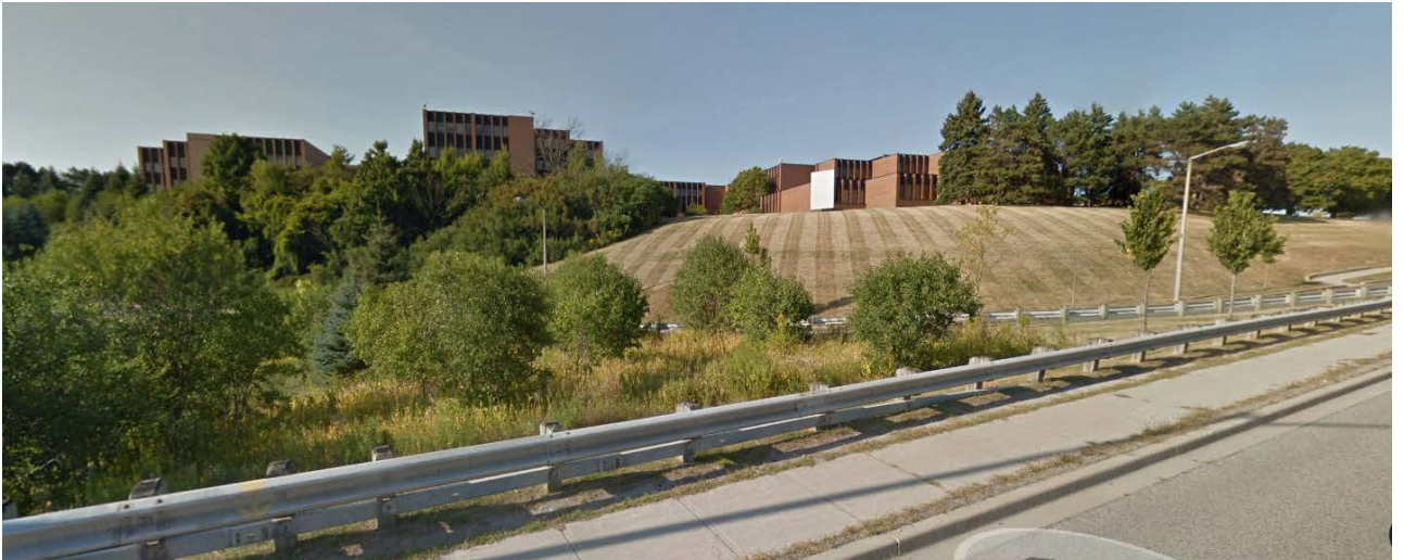
50. 1150 Eglinton Avenue East : viewed from Eglinton Avenue East with the setting of the hilly, well-treed landscape and extensive lawns ( Google Maps )
