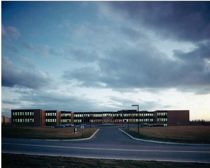
38. IBM Headquarters, North Entry Court 1966-67 : showing the building prior to Phase 2 (Panda Associates, IBMhq-06, NORR Architects, Engineers and Planners)
