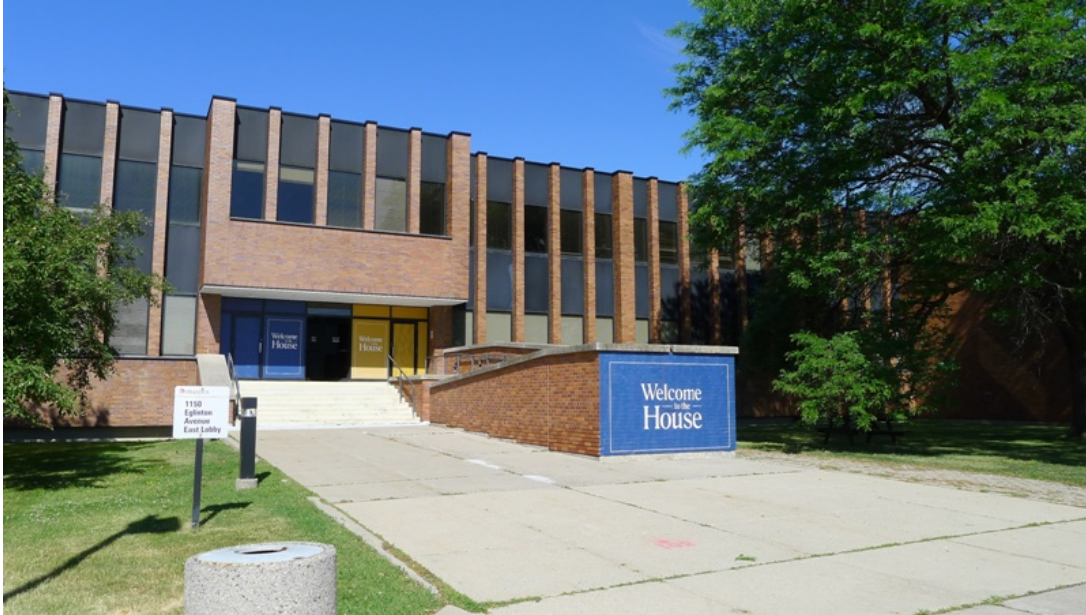
43. East Entry : showing the same arrangement as the north entry with the broad steps, recessed doors and cantilevered bay here modified with a ramp for universal access. The east elevation faces the parking lot but is set back in lawns with mature trees ( HPS, 2016 )
