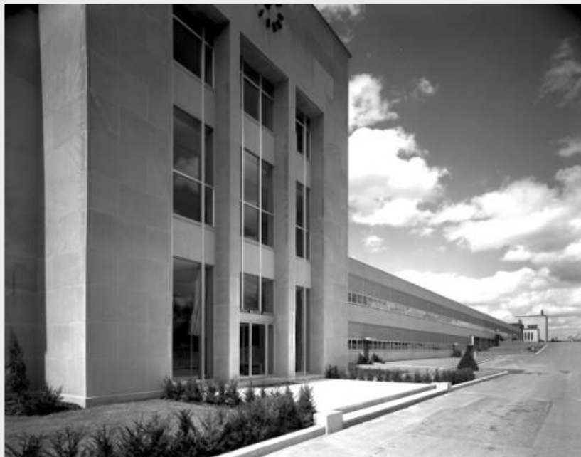
24. IBM Building : showing entry pavilion of the south wing completed in 1954 and looking northwards at the gradual slope in the land where the lower storey emerges to create a two-storey building at the south end. Note the formal landscaping, steps and low corner pylons as well as the unusual detailing which has the window mullions crossing over the stone spandrel panels. ( Canadian Architectural Archives, Panda, 54416-20 )
