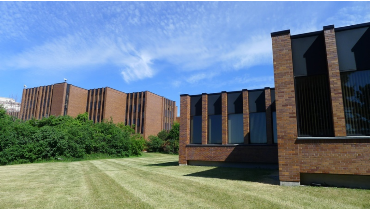
40. IBM Headquarters : looking north-west towards a sequence of landscaped courtyard spaces facing south with the single-storey cafeteria in the foreground. ( HPS, 2016 )
