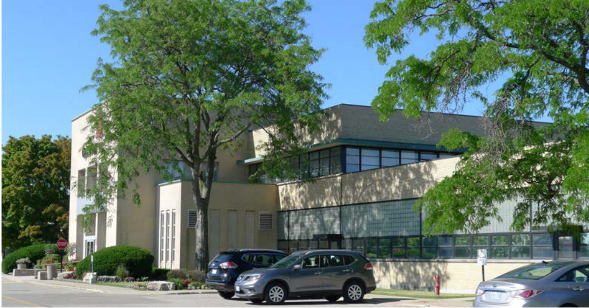
26. IBM/Celestica, north entry pavilion : showing the east elevation of the 1951 portion of the building with the projecting plane over the upper office windows and the horizontal treatment of the wings of the plant space with the bands of buff brick, clear glass and glass block. (HPS, 2016)
