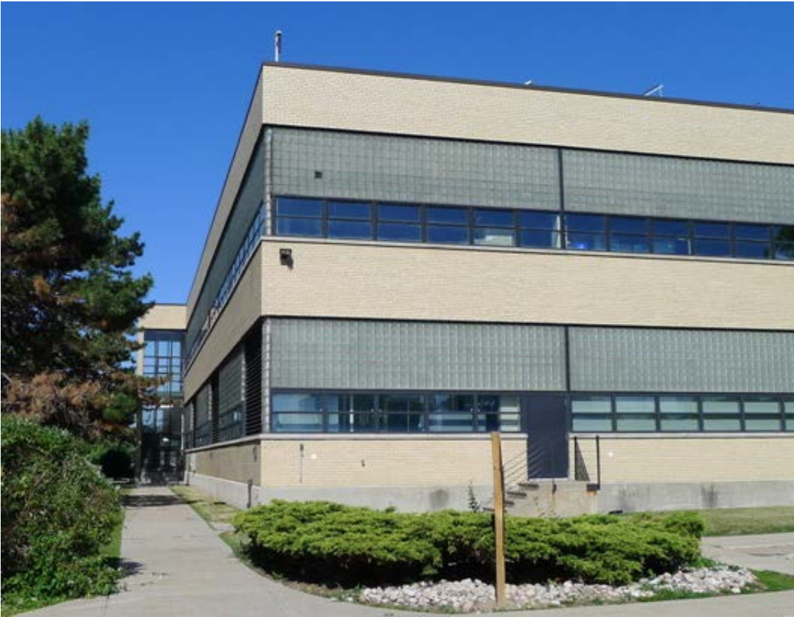
29. IBM/Celestica, East Elevation : showing the south wing completed in 1954, with later entrance and handrail details. (HPS, 2016)
