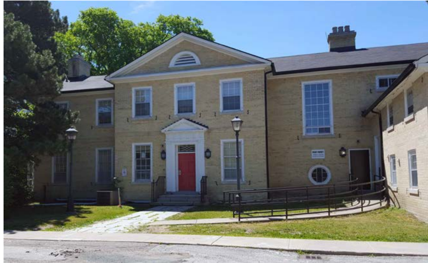
Above: principal (north) elevation, showing the east end with the main entrance; cover: north elevation, showing the west end and the north service wing (Heritage Preservation Services, 2016)
