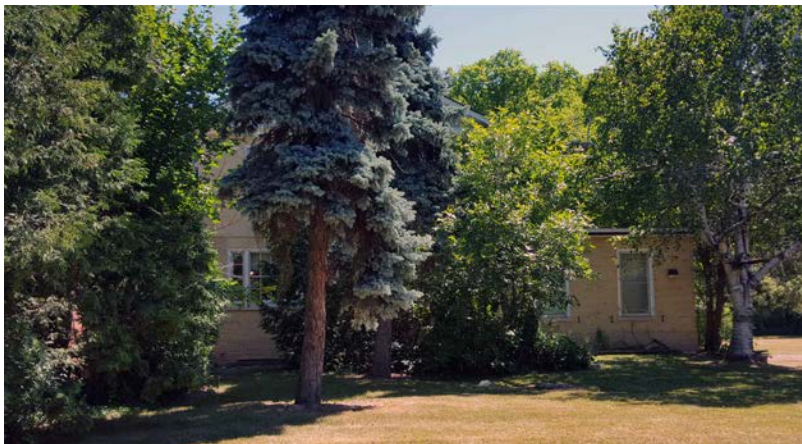
16. Current Photographs, 10 Buchan Court, July 2016: showing the north service wing (top), the east elevation with the open verandah (centre), and the west elevation (bottom) (at the west end of the service wing, the single-storey addition with the red brick is not identified as a heritage attribute) (Heritage Preservation Services).
