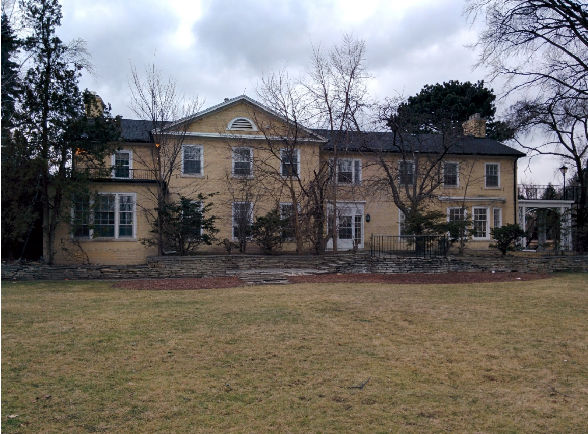
PHOTOGRAPH – SOUTH ELEVATION: 10 BUCHAN CRT
