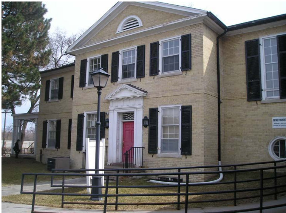
14. Photographs, 10 Buchan Court, 2004 (above) and 2009 (below) : showing the principal (north) elevation before and after the removal of the white paint, and prior to the removal of the louvered wood shutters (Heritage Preservation Services).
