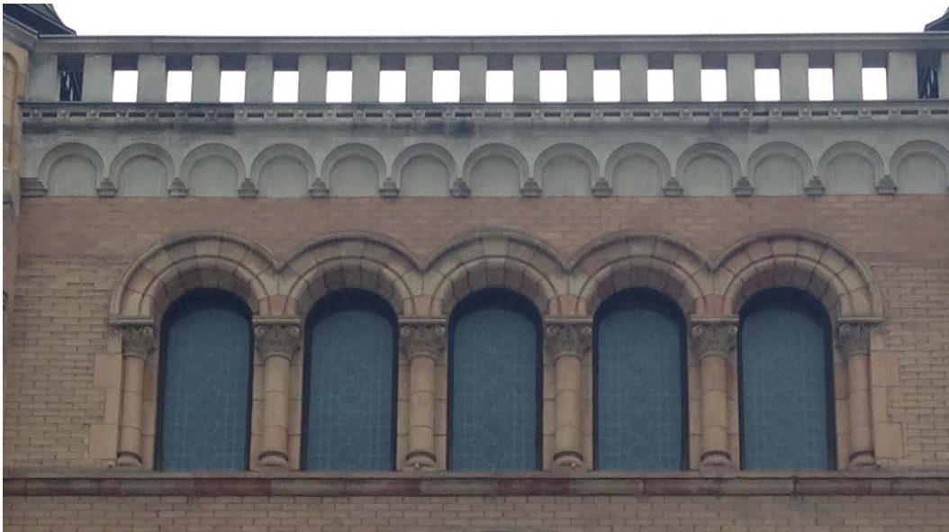
26. 115 Bond Street: showing the arcade at the third level above the tympanum with its row of colonettes and composite capitals and above the restored parapet of arches and balustrade (HPS, 2016)
