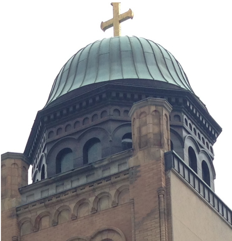
27. 115 Bond Street: showing one of two original octagonal drums on the towers with its richly detailed cornice and pairs of windows, as well as the octagonal turrets terminating the piers of the tower. Note the arches of the parapets and the brick colonettes with their capitals. The new copper dome with its bell cast curve and the cross were part of the 1980s renovations (HPS, 2016)
