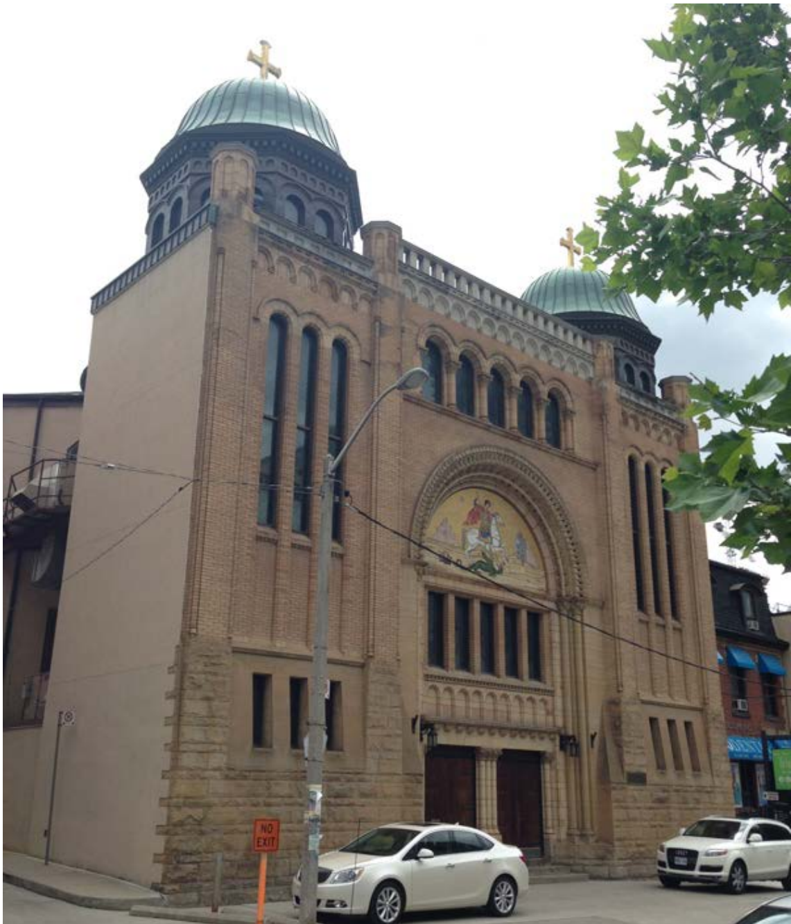
21. 115 Bond Street, Saint George's Greek Orthodox Church (former Holy Blossom Synagogue): showing the west elevation post the 1982-7 renovations which included the addition of the mosaic in the tympanum and the replacement of the original onion domes on the two drums of the towers and the removal of the four small onion domes on the piers (HPS, 2016)
