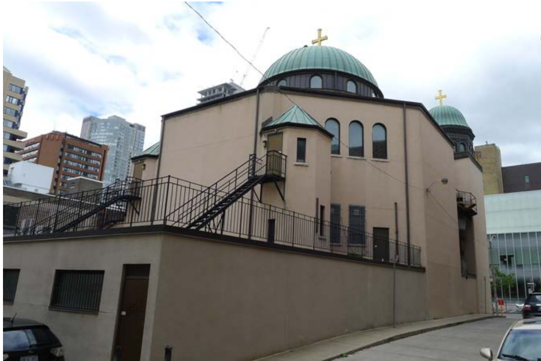
19. 115 Bond Street: showing the rear north and east elevations, the principal octagonal volume of the domed prayer space, the two small towers for the spiral stairs and the 1958 one-storey extension. (HPS, 2016)
