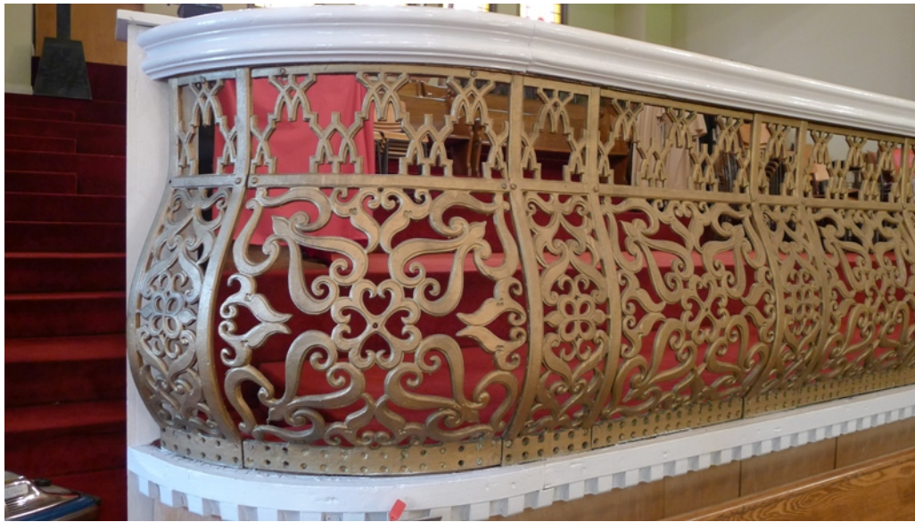
35. 115 Bond Street, Balustrade: showing the gallery balustrade composed of pressed metal panels in an arabesque design. (HPS, 2016)
