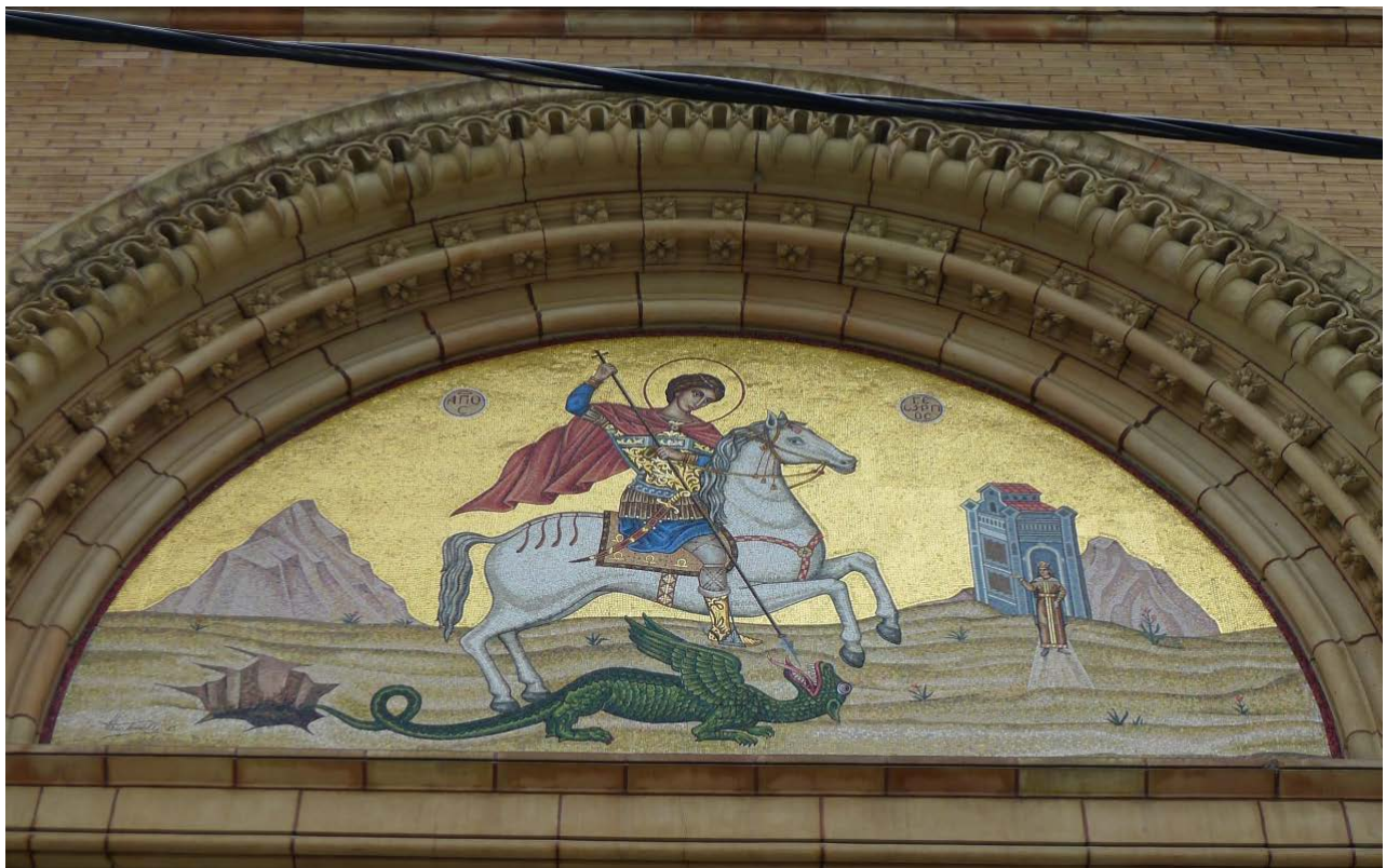
25. 115 Bond Street: showing the rich variety of original carved details of the great arch with the 1987 mosaic of Saint George slaying the dragon by Sirio Tonelli in the tympanum (HPS, 2016)
