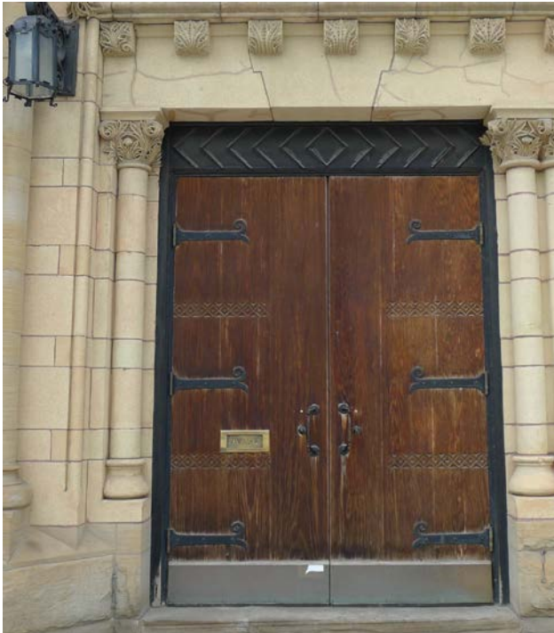
29. 115 Bond Street: showing the left-hand pair of the new set of doors installed prior to the 1980s renovations (HPS, 2016)
