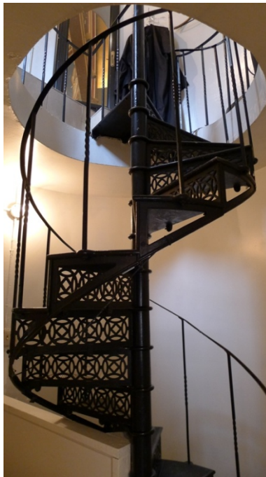
40. 115 Bond Street, Spiral Stairs: showing the original spiral stairs on the east side of the church providing access between the sanctuary and the offices. (HPS, 2016)
