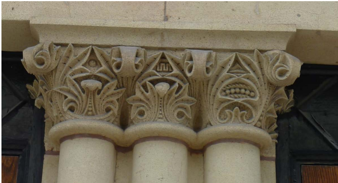
24. 115 Bond Street: showing the intricate and varied details of the carving of the three Romanesque capitals between the two entry doors. (HPS, 2016)
