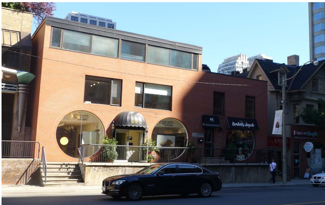
View of west elevation of the building complex. Shown is the portion with the municipal addresses 45-49 Avenue Road.
