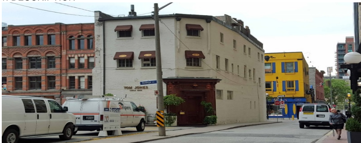
Above: north (left) and west (right) elevations of 40 Colborne Street; cover: south (right) and west (left) elevations (Heritage Preservation Services, 2016)
