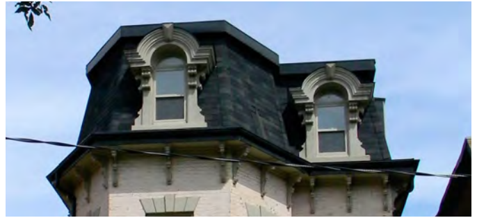
Figure 10: Mansard roof in the Garden District HCD
