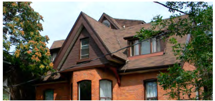
Figure 11: Gabled roof in the Garden District HCD
