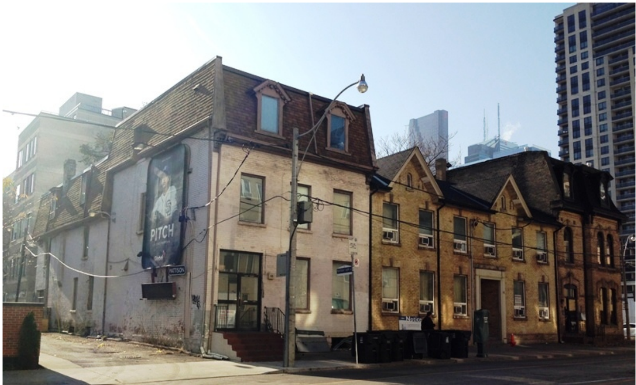
Photograph of the block on the south side of Shuter Street showing the north elevations as well as the east elevation of 85 Shuter Street facing the laneway (HPS, 2016)
