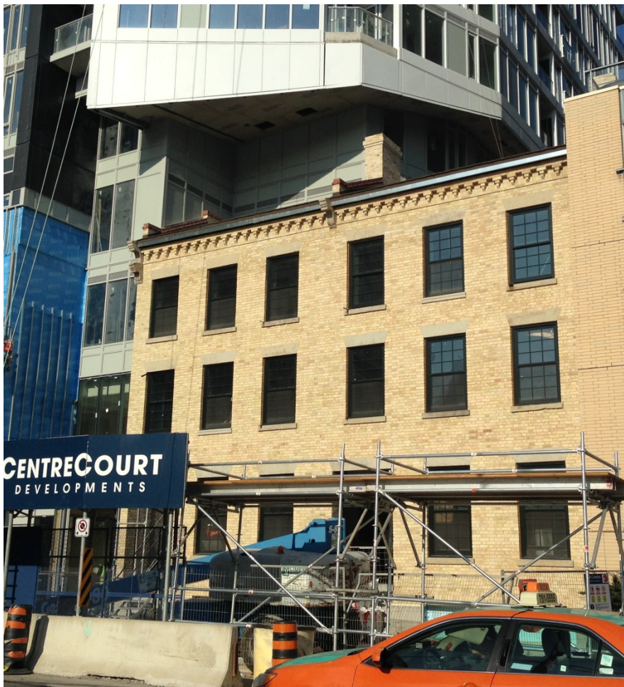
15. 68 and 70 Shuter Street following restoration and new development. (HPS, 2016)
