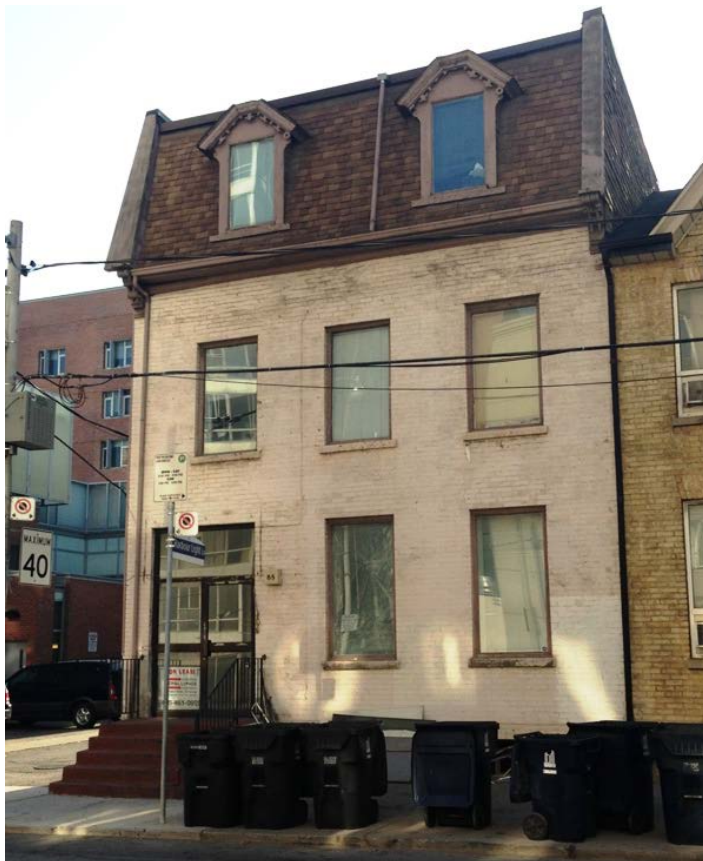
85 Shuter Street, showing the north elevation (HPS, 2016)
