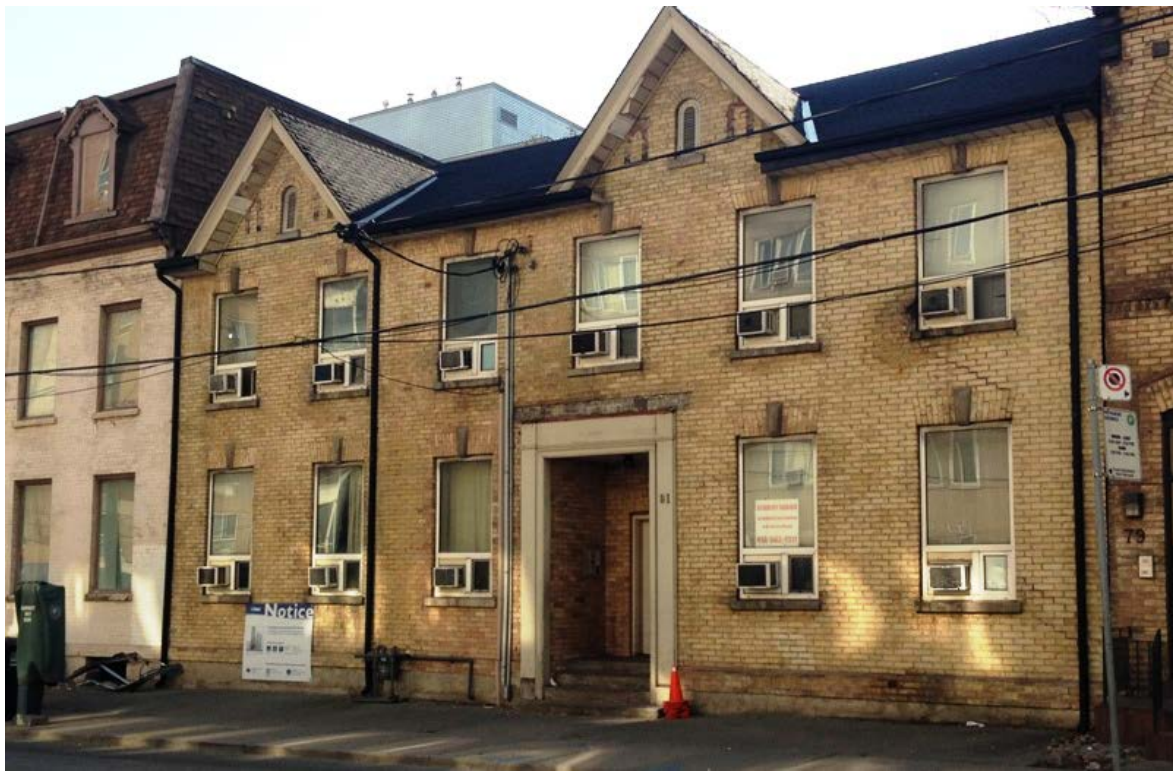
20. 81 Shuter Street, North elevation: showing the current condition of the former 83 and 81 Shuter Street, now united with a single entrance and the replacement to the left of the entrance with a window whose proportion matches the existing windows. (HPS, 2016)
