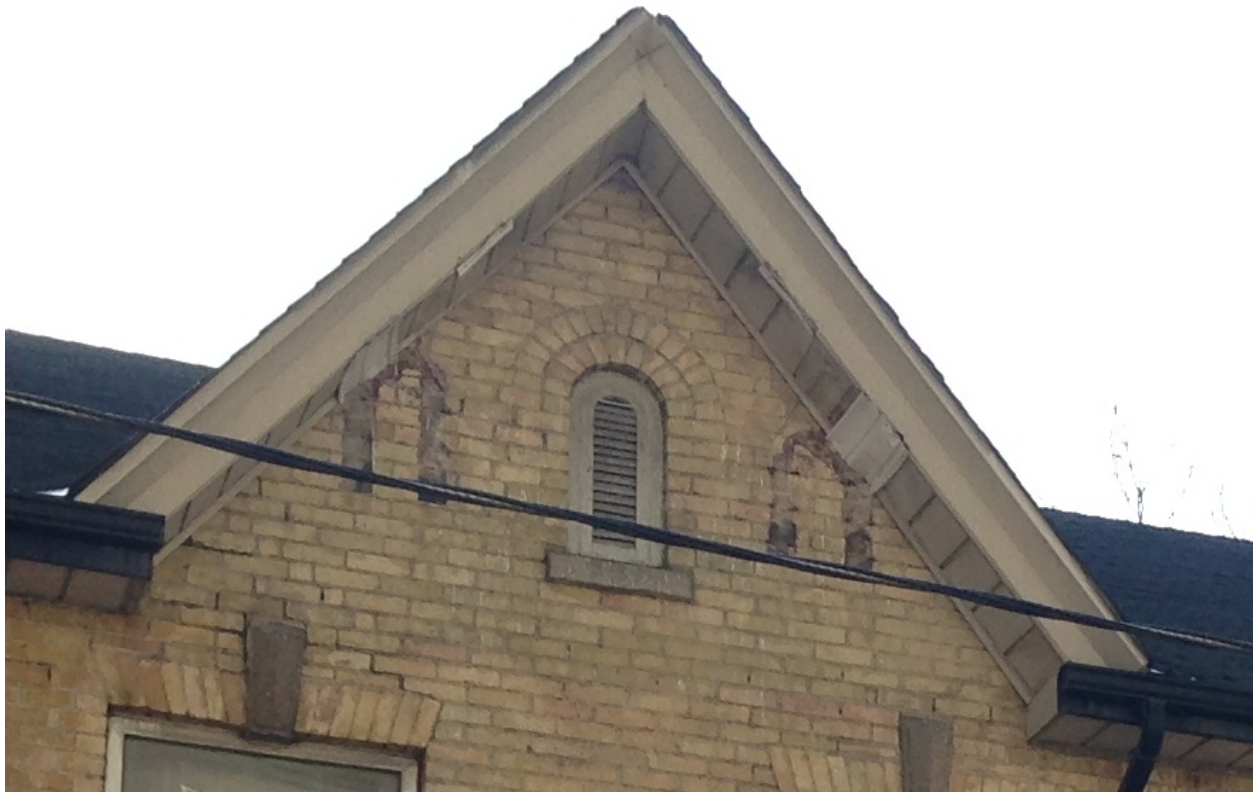
25. 81 Shuter Street, North elevation, gable detail: showing location of former wood brackets. (HPS, 2016)
