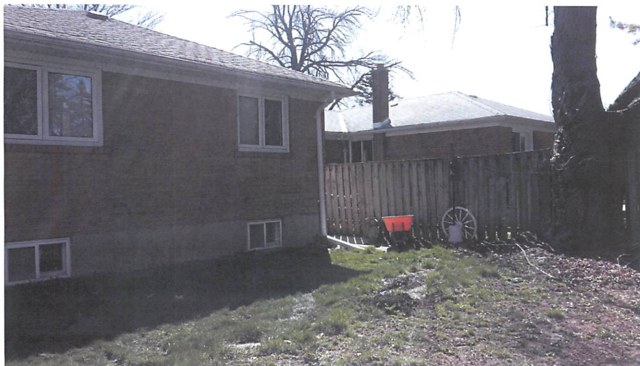
238 Livingston Road- Photo 1 Rear Yard
