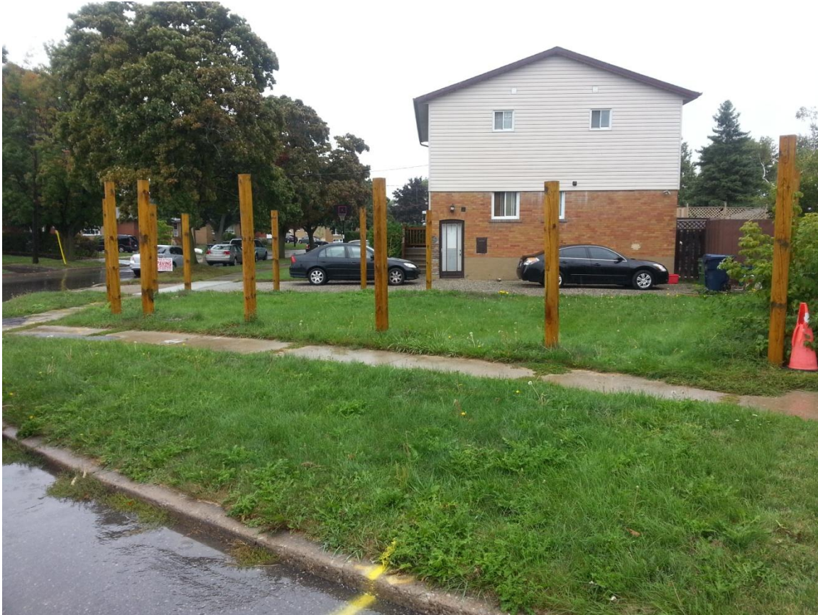
Existing Fence posts at 9 Frolick Crescent looking north/east.
